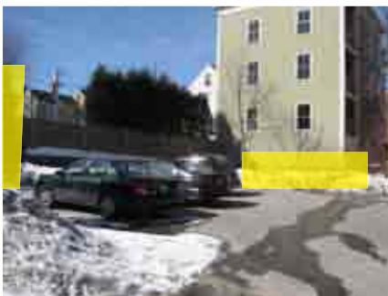
Large trees are overgrown and should be trimmed in order to allow proper drying and avoid future maintenance costs.
