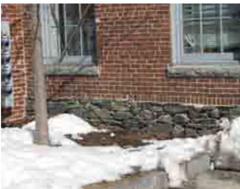
Stone foundation in this one area is in good shape.
