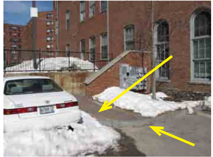
Granite curbing and brick walkway appear newer.
