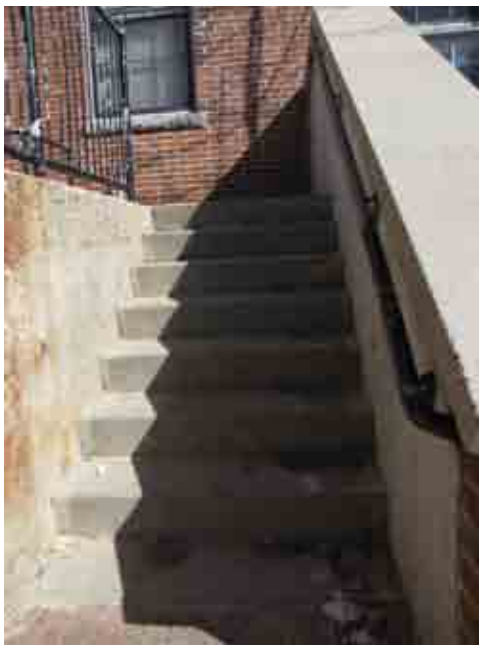
Concrete steps in good shape
