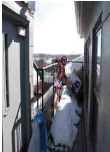
Snow blocking the egress and maybe the cause of water damage in the stair tower.
