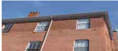
There is a difference in brick and mortar on the third floor exterior. This comes from an addition to the building, date unknown, to expand the third floor.
