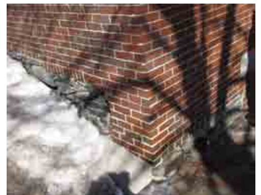
Stone foundation in this one area should have attention given to the connection between stone and brick.
