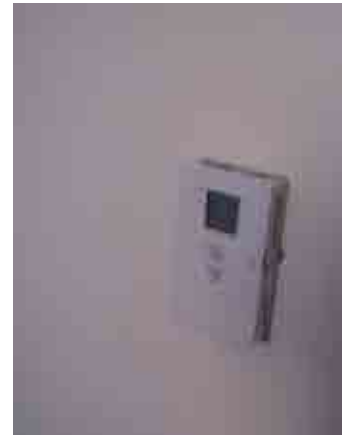
Electronic thermostats in units
