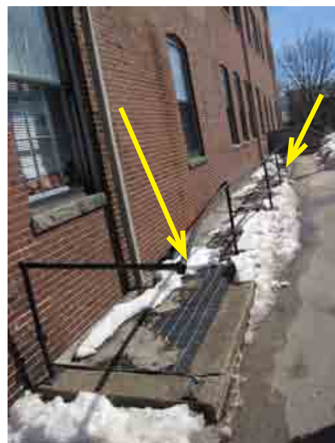
Area in need of fixing or egress area for new sublevel spaces.
