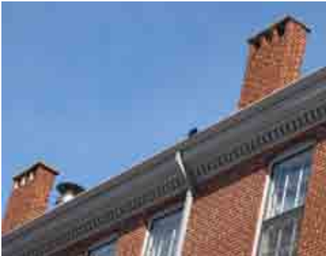
The chimneys appear to be in good shape.
