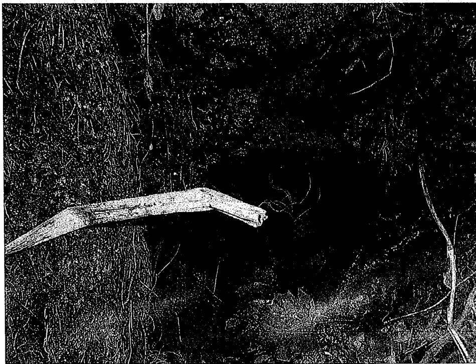
Photo 6 – Non-Functioning 11" Diameter Drain Tile at Bottom of Dam
