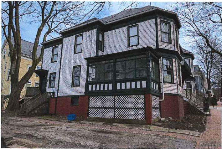
PHOTO OF THE EXISTING BUILDING
