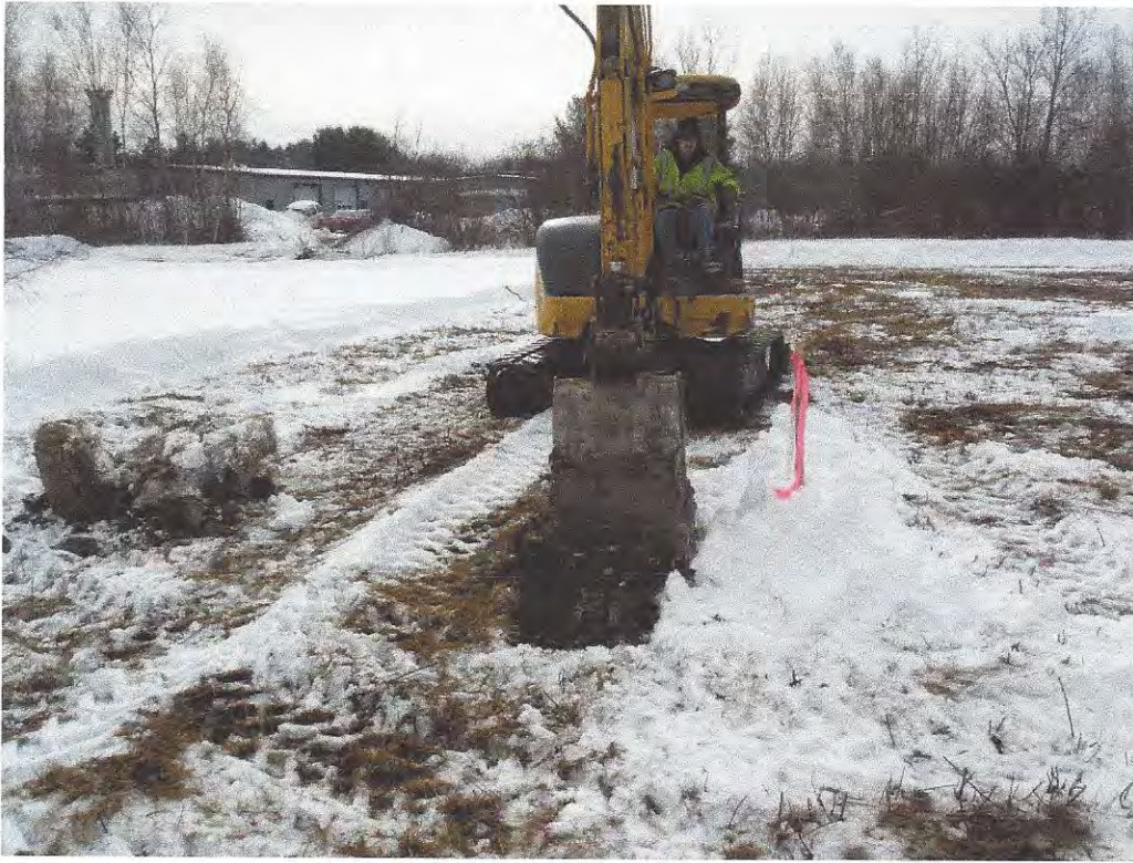
View of excavator near edge of upland
