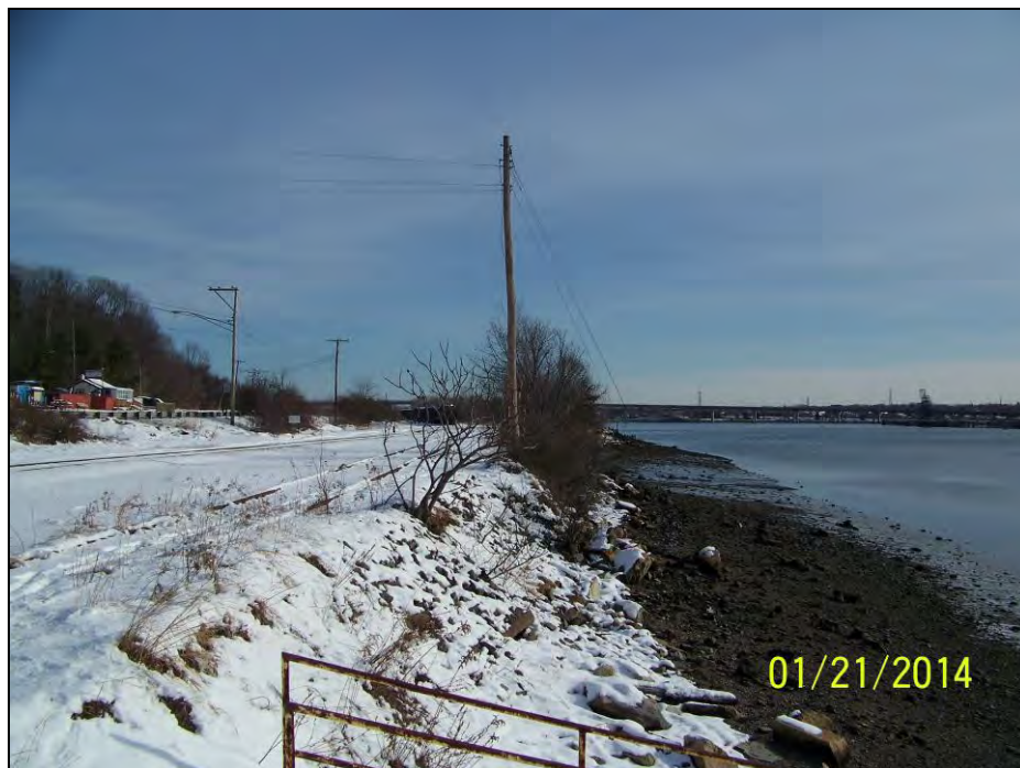
Figure 5 – Picture of the Fore River waterfront at the west end of the site near Cassidy Point Drive shows intertidal areas as evidenced by the lack of snow and ice within the tidal reach, and rock stabilization.
