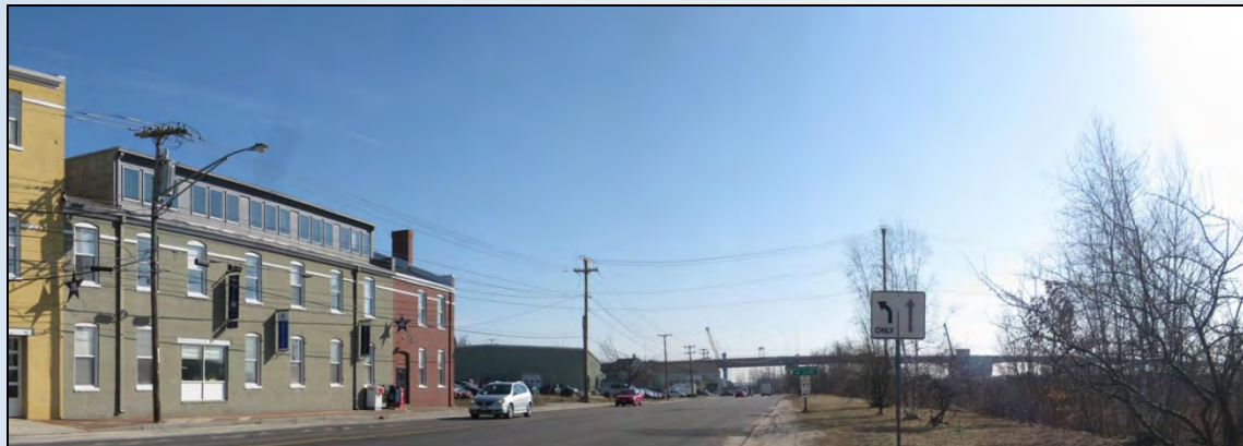
view east existing
