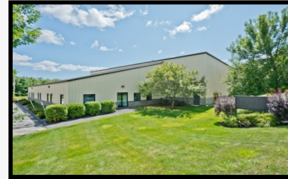
921 Riverside Street, Portland 25,000 SF
