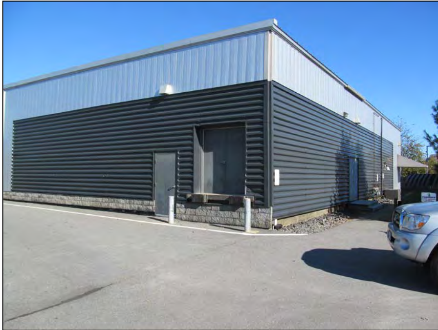
PHOTO 21 – AT&T Store & Planet Dog Building (Year Built 1981)
