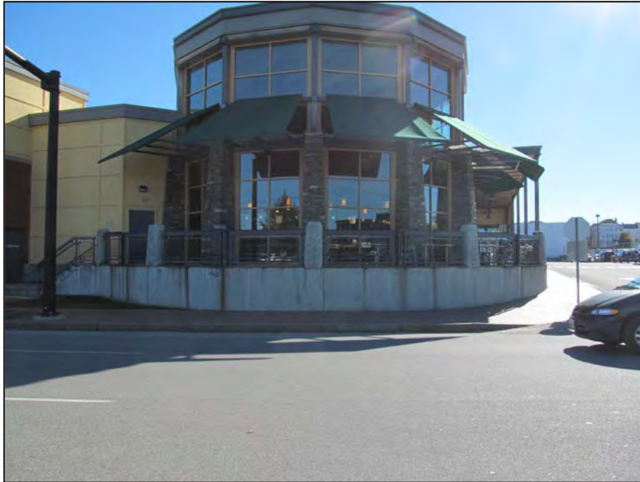
PHOTO 23 – Whole Foods Building (Year Built 2006)
