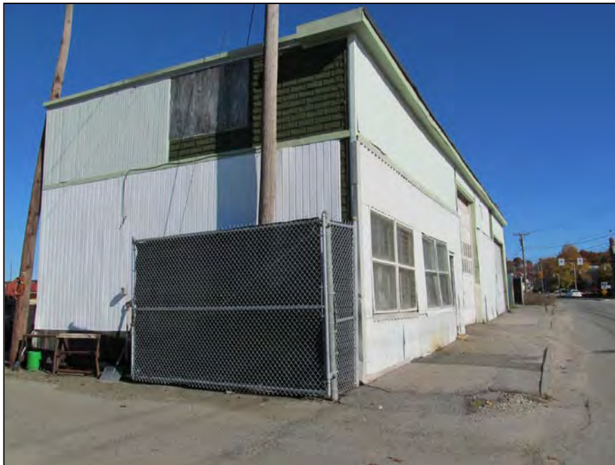
PHOTO 18 – Warehouse Construction Yard Area (Year Built 1940)
