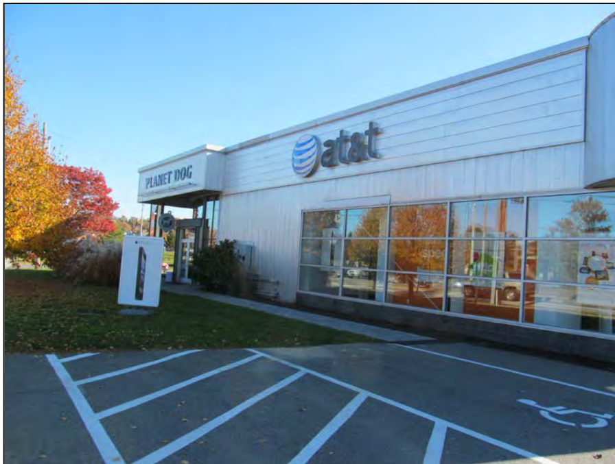
PHOTO 22 – AT&T Store & Planet Dog Building (Year Built 1981)
