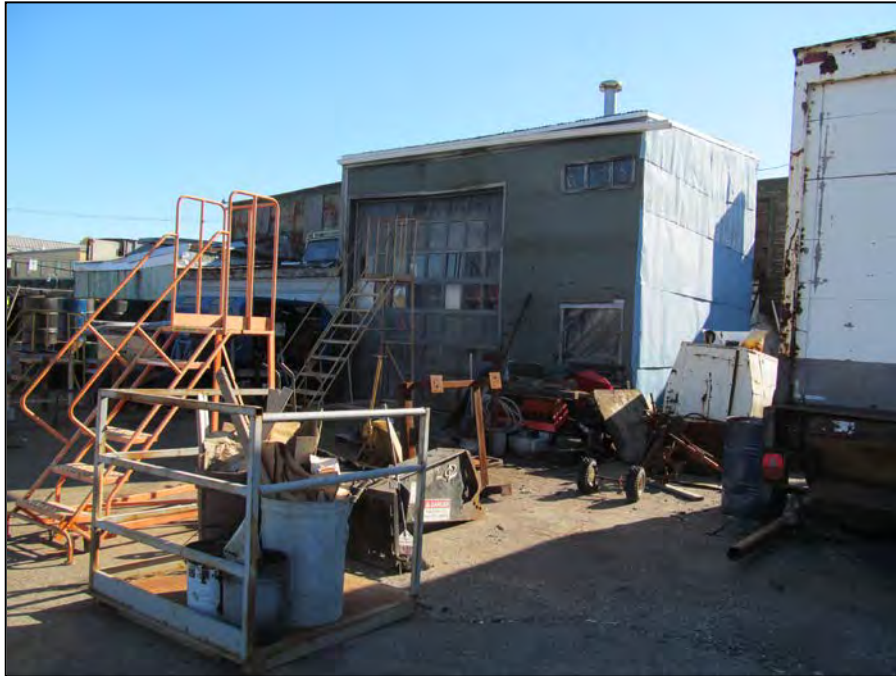
PHOTO 17 – Warehouse Construction Yard Area (Year Built 1940)
