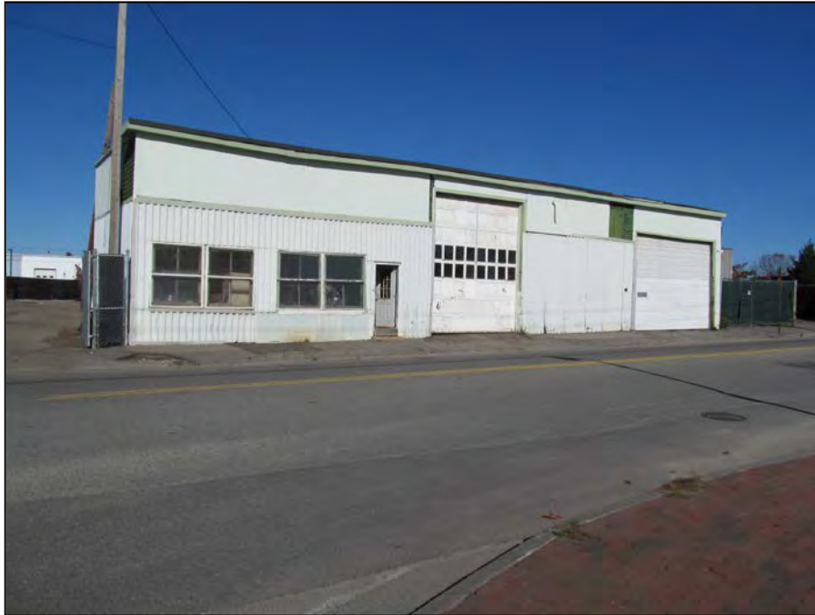
PHOTO 19 – Warehouse Construction Yard Area (Year Built 1940)
