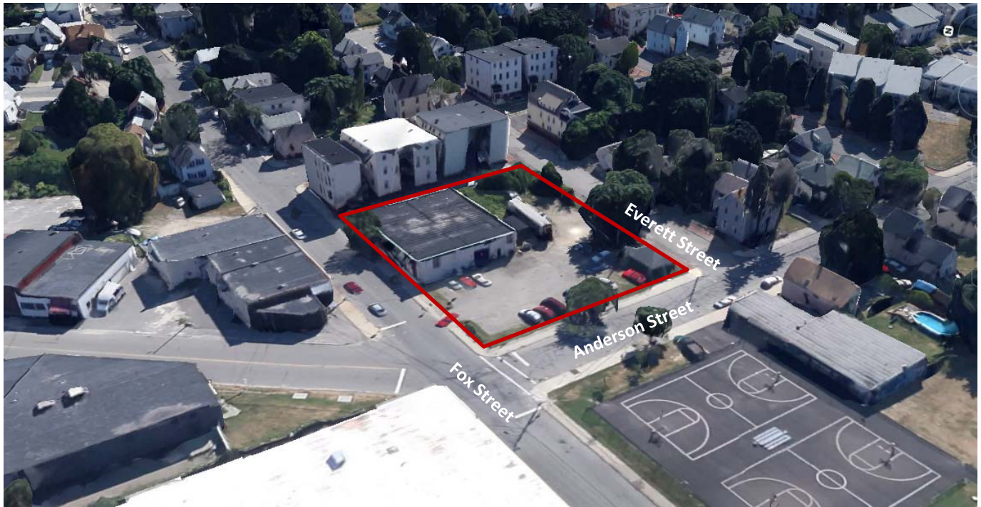
Figure 1: 89 Anderson Street site
