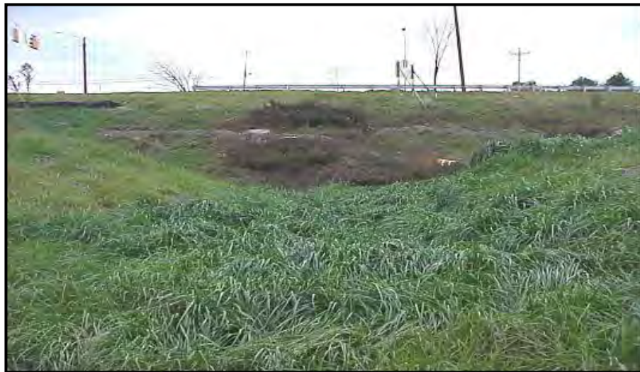
A WELL-STABILIZED VEGETATED SWALE SHOWS LITTLE SIGNS OF EROSIVE VELOCITIES OR FLOWS. THIS SWALE ALSO FUNCTIONS AS A POND SPILLWAY
