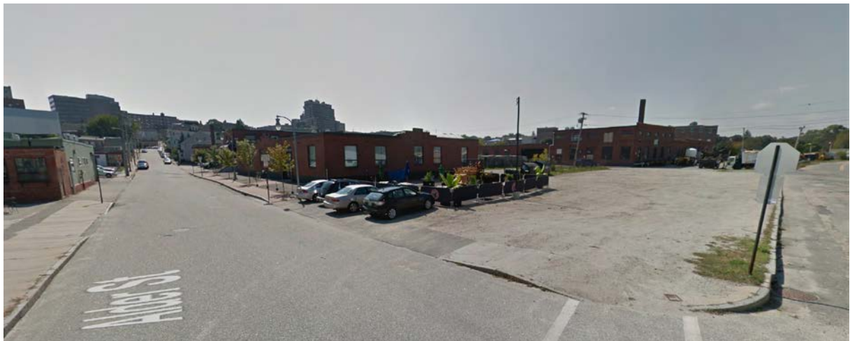
View of Bayside Bowl Corner of Alder Street and Kennebec Street
