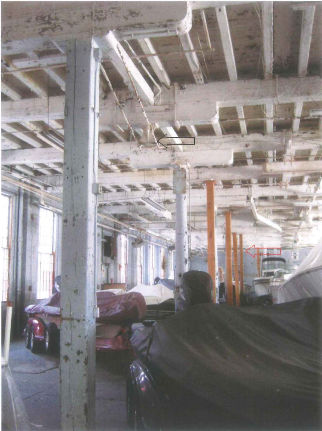
Photo 2-2: Interior photo, building 2 taken from the ground floor. Note added posts, king post truss.
