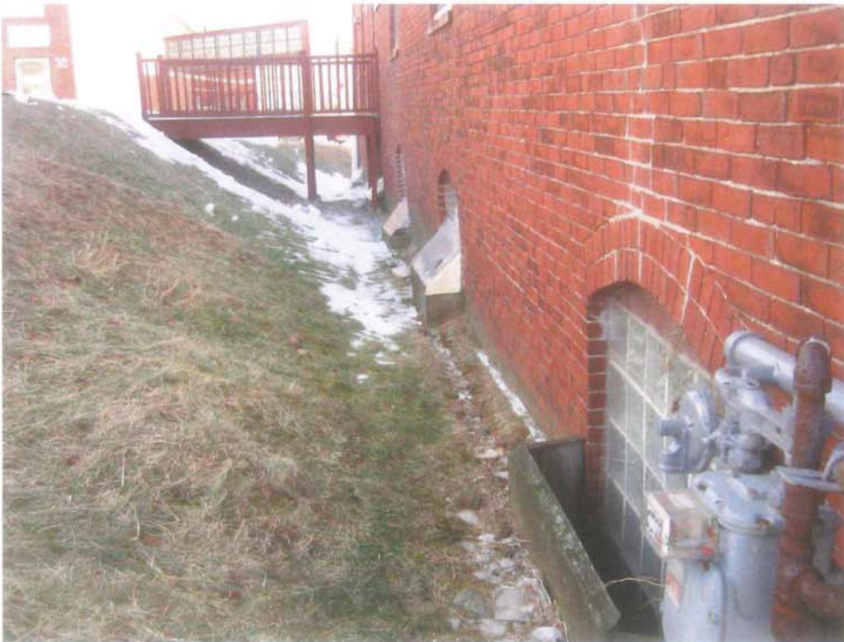
Photo 11-4: Window wells and embankment at north wall.
