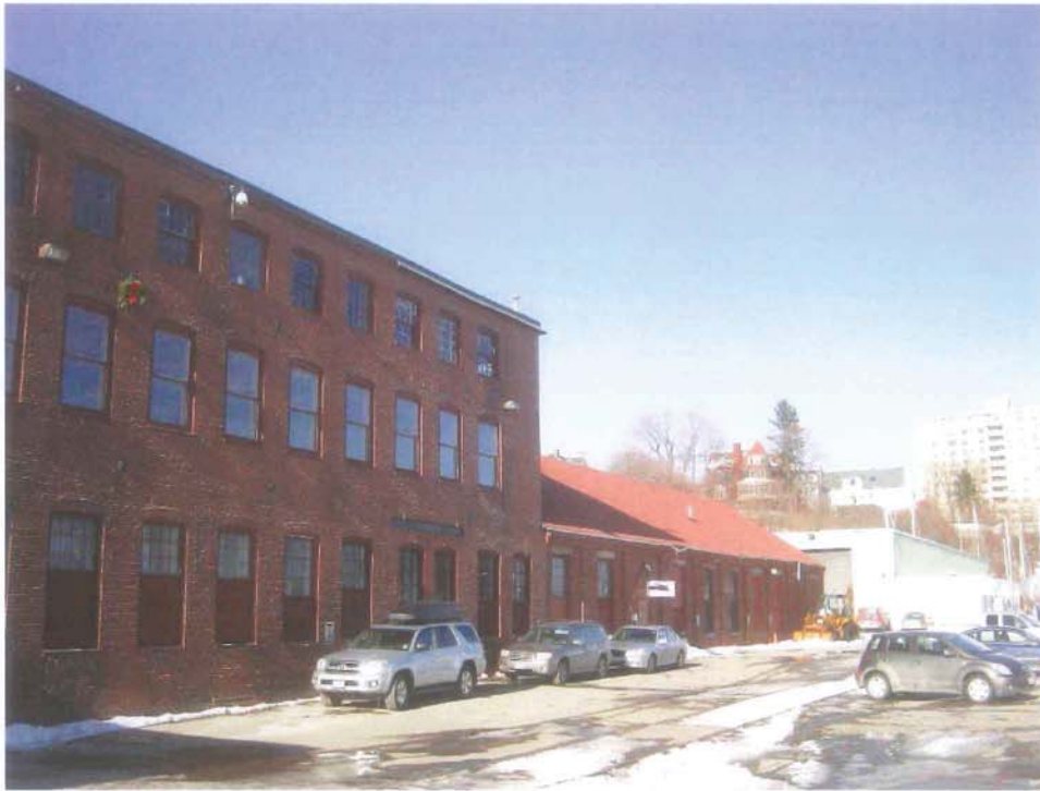
Photo 6B-1: Buildings 6A (left) and 6B (right).
