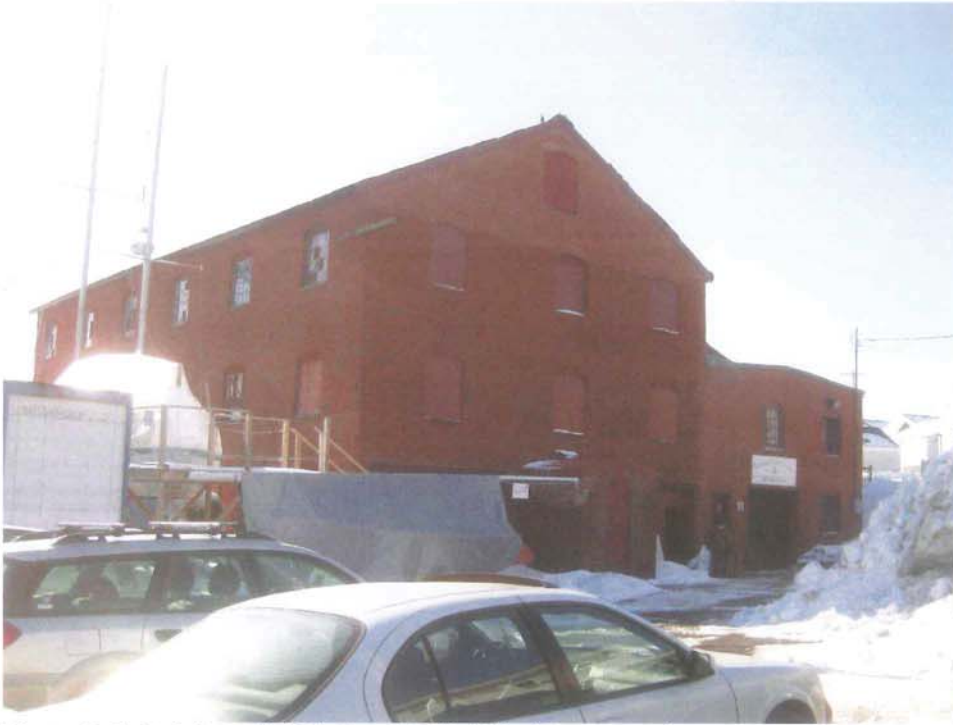
Photo 11-1: Buildings 11 (right) and 12 (left) looking at southeast corner.
