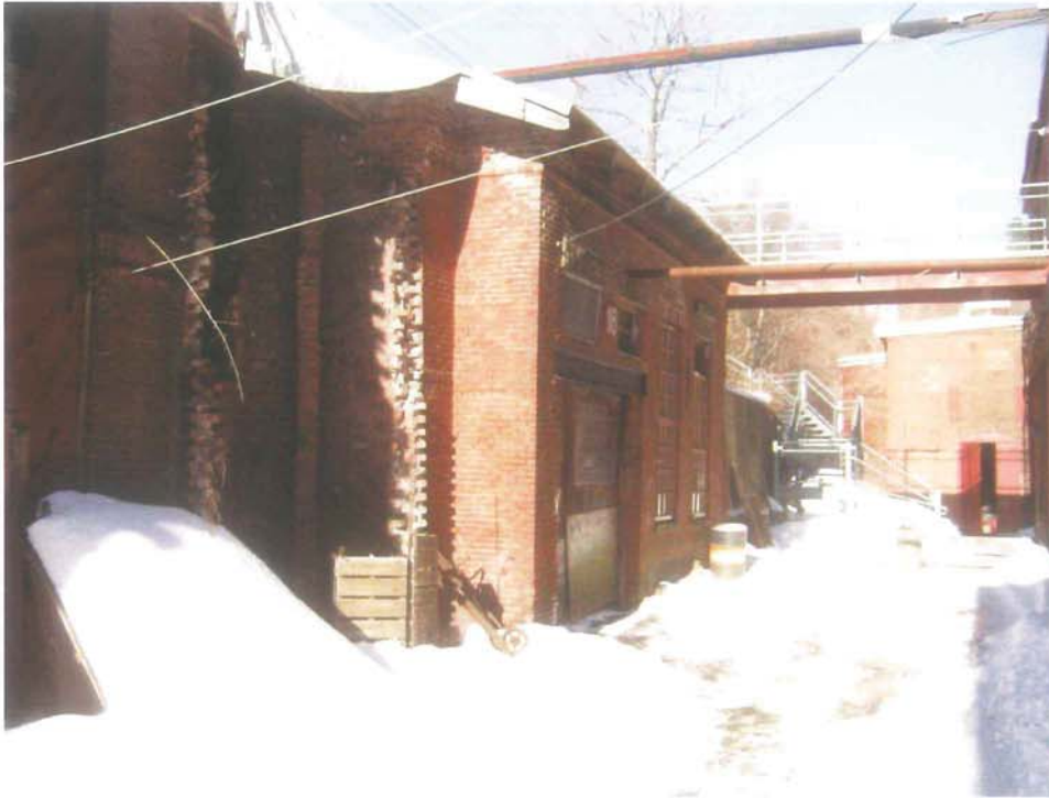
Photo 16-1: Exterior view of blacksmith shop/Building 16.
