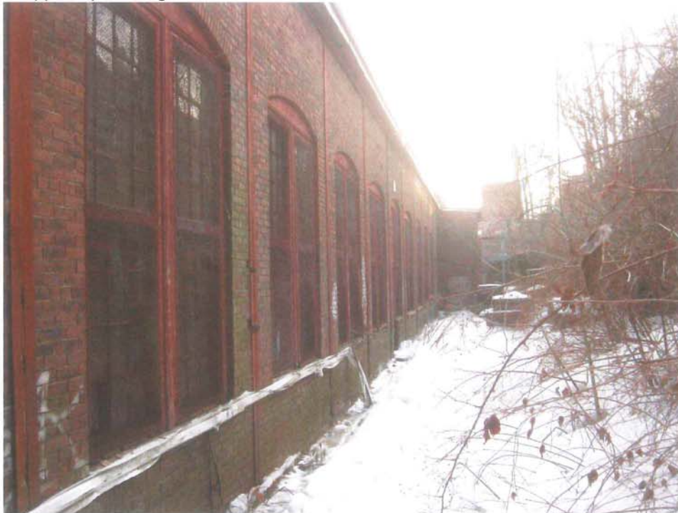
Photo 4-2: Exterior of Building 4, North Side.
