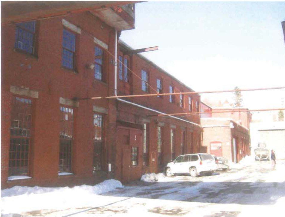
Photo 3-1: Exterior view of Building 3
