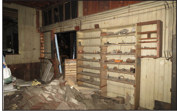
Current view of the lab/office space.
