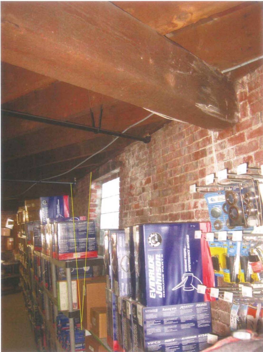
Photo 11-3: Bowed north wall retaining embankment (lines added for emphasis).
