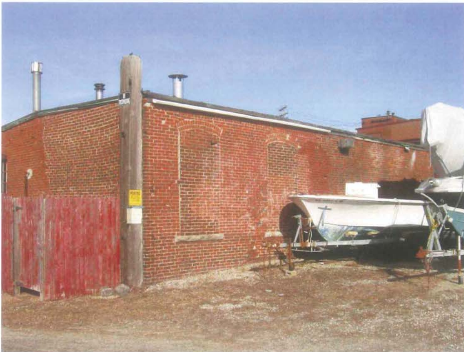
Photo 10-2: Exterior view of Building 10.
