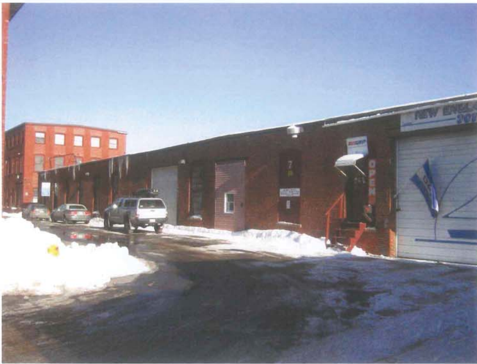
Photo 7-2: North elevation of Building 7.
