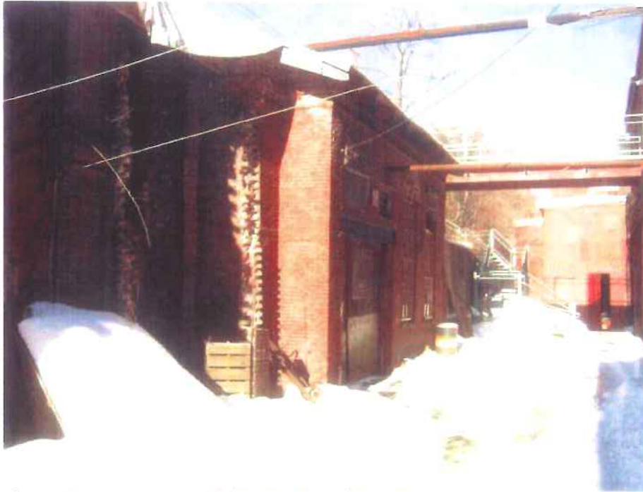
Photo 16-1: Exterior view of blacksmith shop/Building 16.
