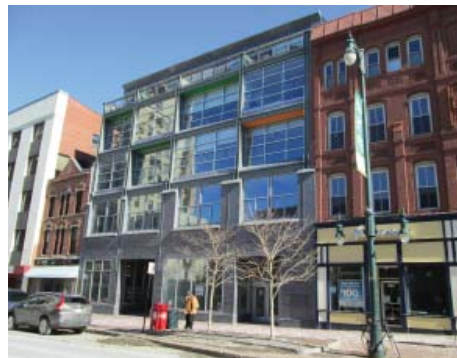
Base/Middle/Top, Change of facade planes, Recessed entry, Storefront, Window details create scale, Stepback, Overhang Cornice line
