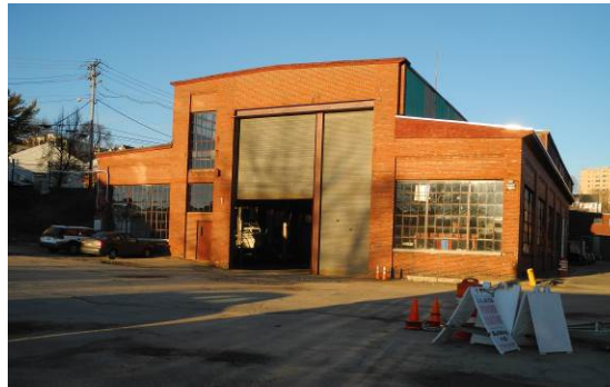
Building 1 – Erecting Shop, west Elevation
