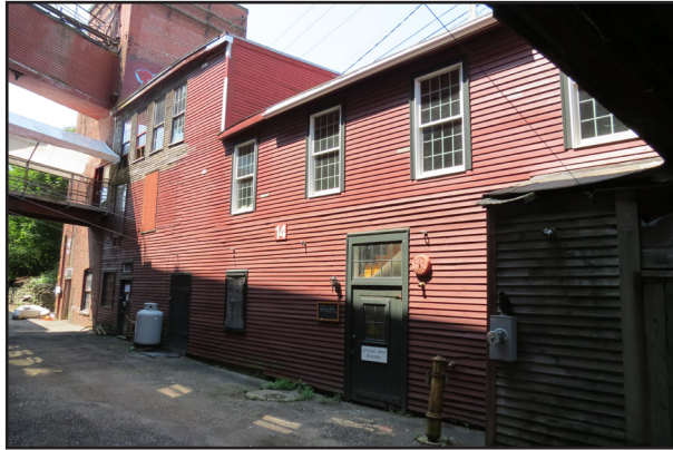
Building 14: Drafting Room and Storehouse Construction Date: 1858-64
