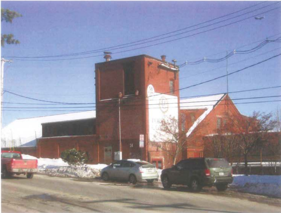
Photo 58-1: 58 Fore Street Vault/Tower structure viewed from Fore Street.
