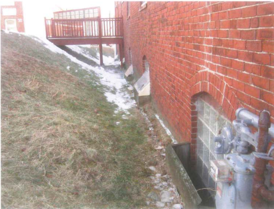
Photo 11-4: Window wells and embankment at north wall.
