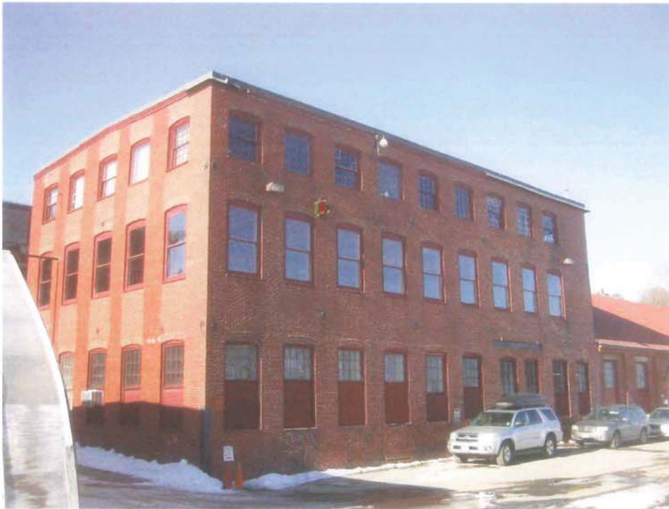
Photo 6A-1: Building 6A exterior view.
