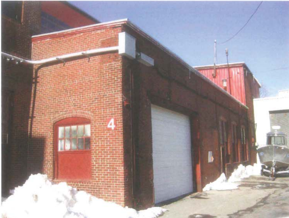
Photo 4-1: Exterior of Building 4. Note a majority of the south and east faces of the building are wrapped by Building 5.
