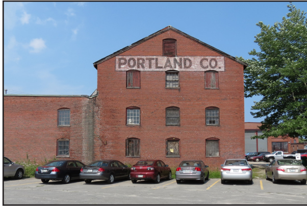
Building 12: Pattern Storehouse Addition Construction Date: 1895
