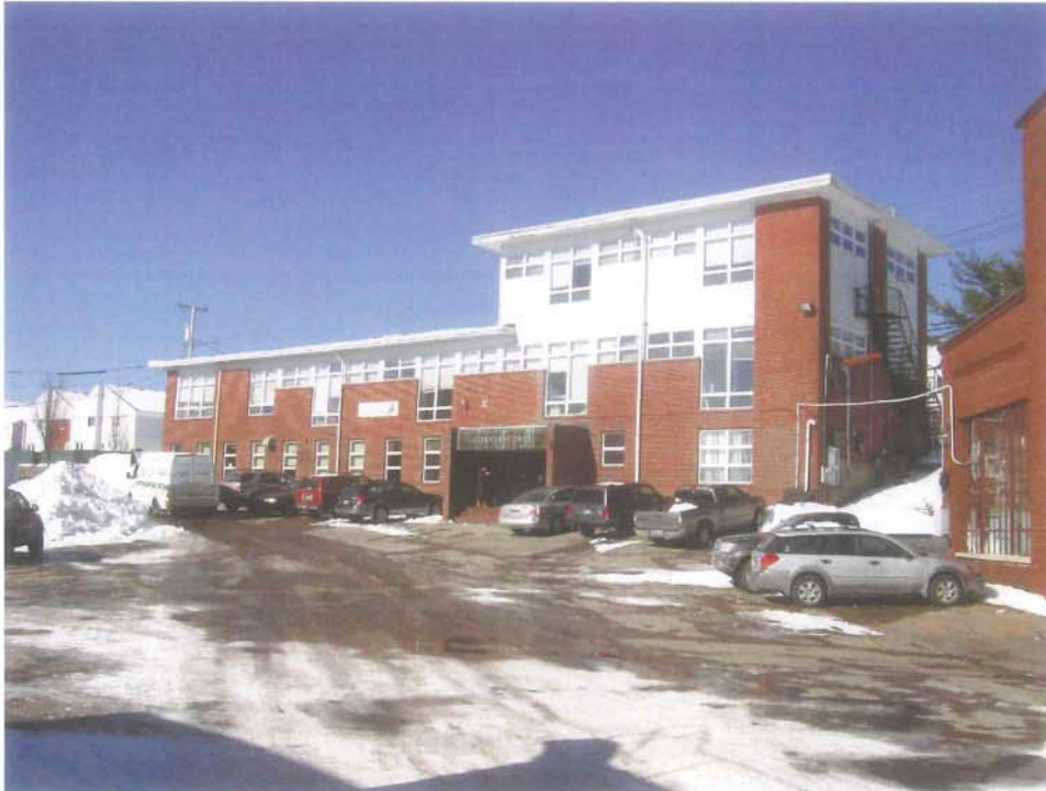
Photo 30-1: Southwest elevation of building 30.
