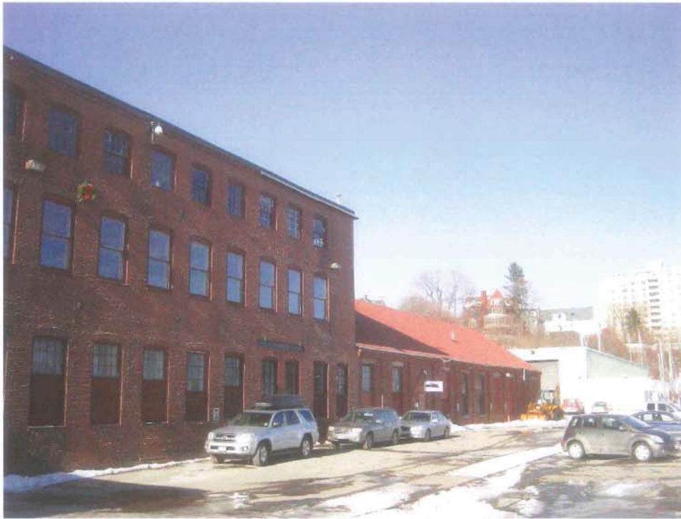
Photo 6B-1: Buildings 6A (left) and 6B (right).
