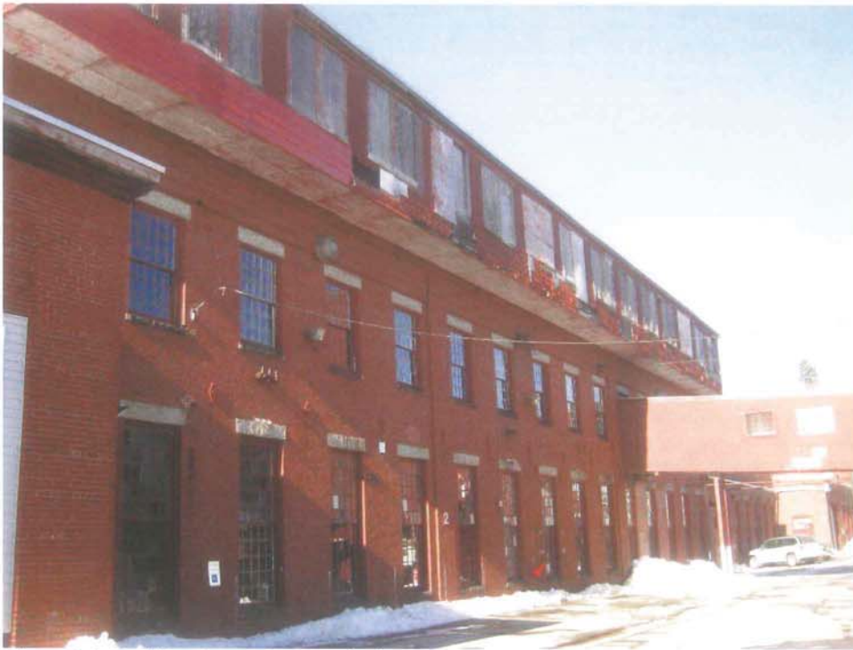
Photo 2-1: Building 2 exterior south elevation.
