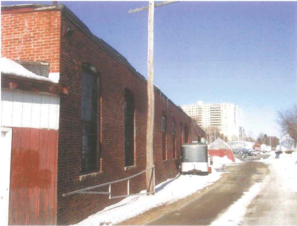
Photo 7-1: South elevation of Building 7.
