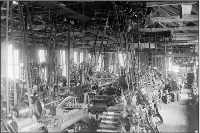
Interior of the machine shop. Courtesy of the Maine Historical Society.
