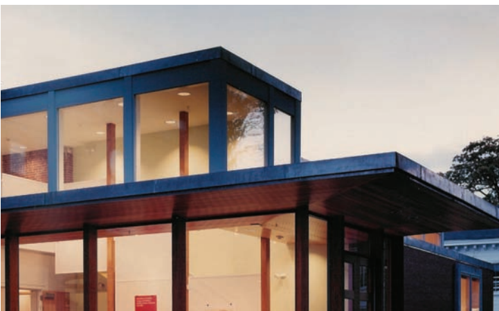
Flashing and trim details should have clean lines and carefully articulated edges. -Waynflete School Arts Center by Scott Simons Architects.
