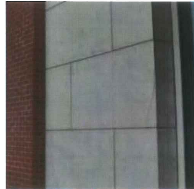
24" x 48" Arriscraft Adair Limestone Anchored Dimensional Stone Vertical Running Bond Installation
