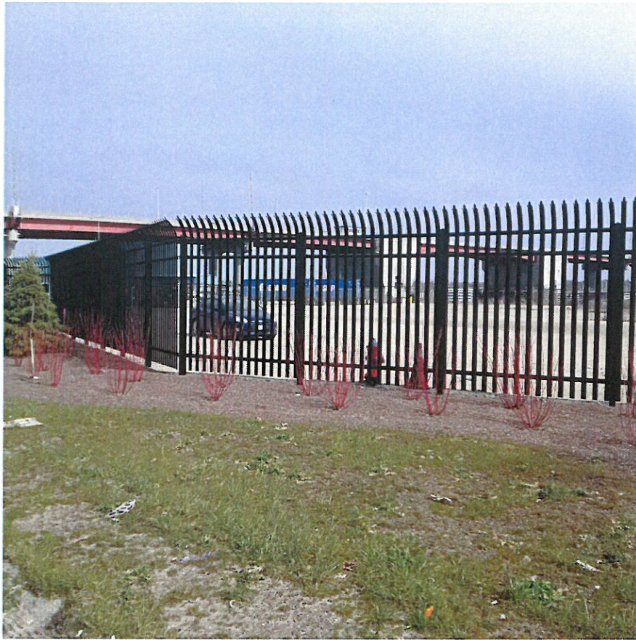
Landscaping Along Fence (winter conditions)
