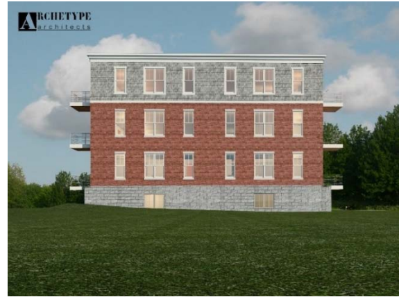
Building 1 from Stevens Avenue
