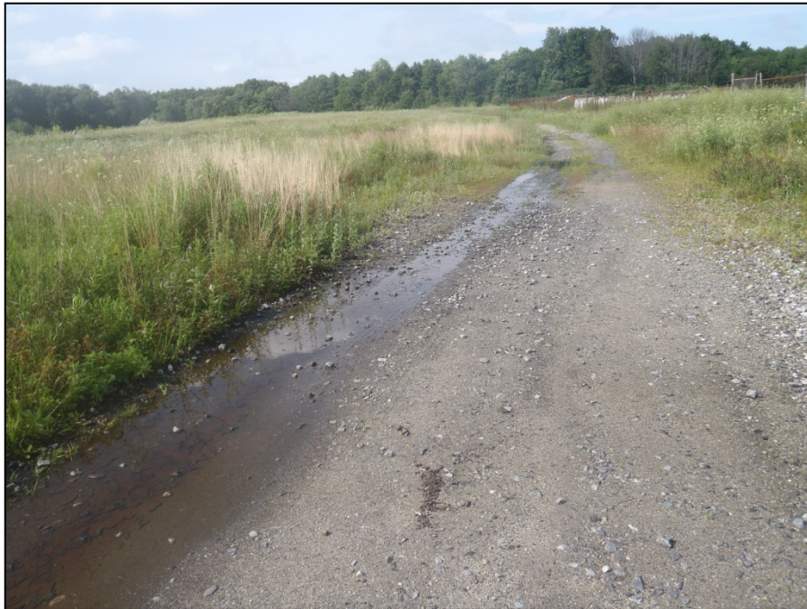
PHOTO 4 – Gravel drive on the site. Looking northerly.
