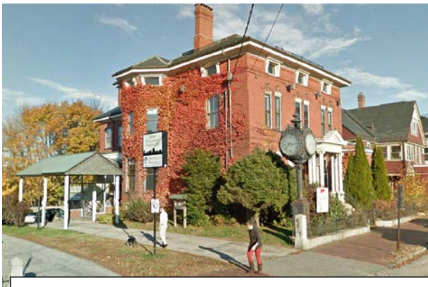
Figure 2: Existing Structure on Congress Street
