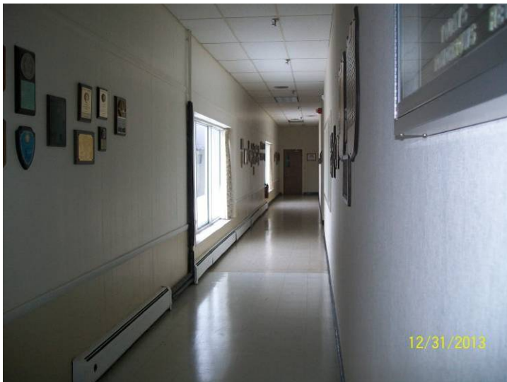
15. Image showing conditions typical of the interior of the Site building.
