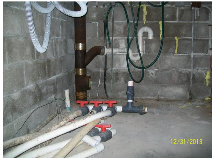
12. Image showing decommissioned pool chemical storage room in northeast corner of pool room.
