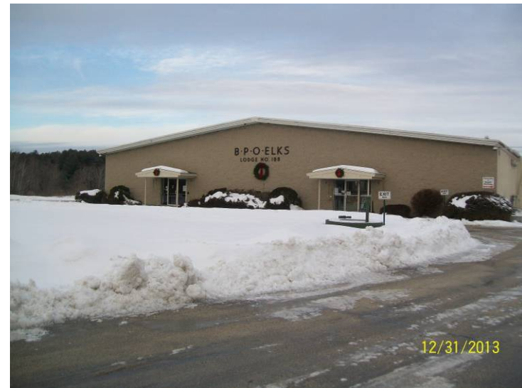
2. Image showing Site building, view facing north from entrance driveway.
