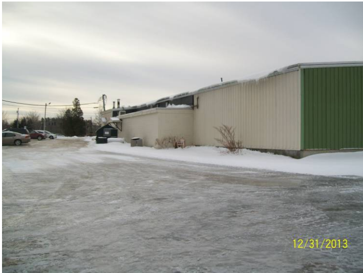
9. Image showing eastern side of Site building, view facing south.
