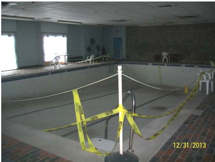
11. Image showing pool room in northwest portion of the Site building.
