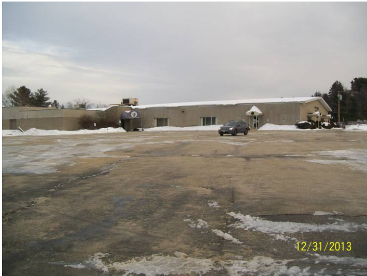
1. Image showing the Site, view facing northeast from western side parking lot.
