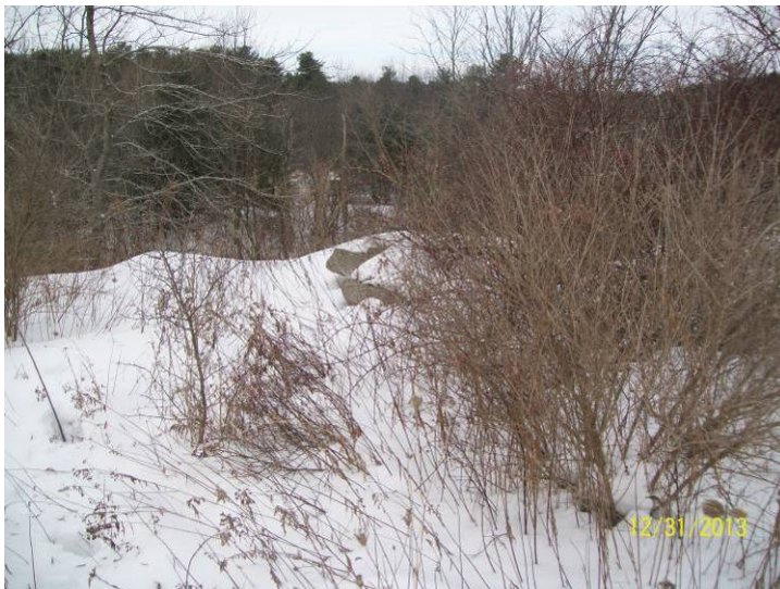
7. Image showing concrete in debris piles.
