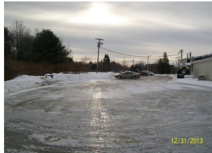
10. Image showing ice covered parking area on eastern side of Site, view facing south. Note disposal (trash and oil) receptacles.
