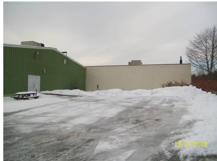
8. Image showing eastern side of Site building, view facing west.
