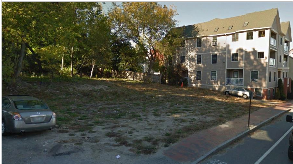
Figure 2: 161 York Street Site
