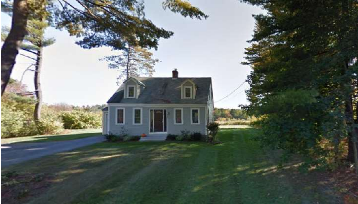
Address: 1646 Westbrook Street
