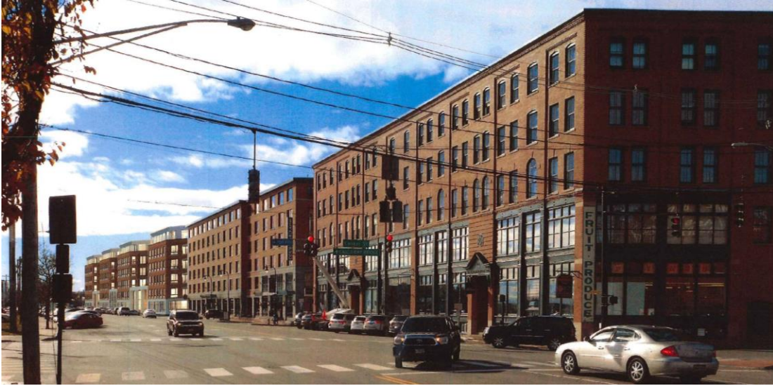
Looking west on Commercial Street toward proposed development
