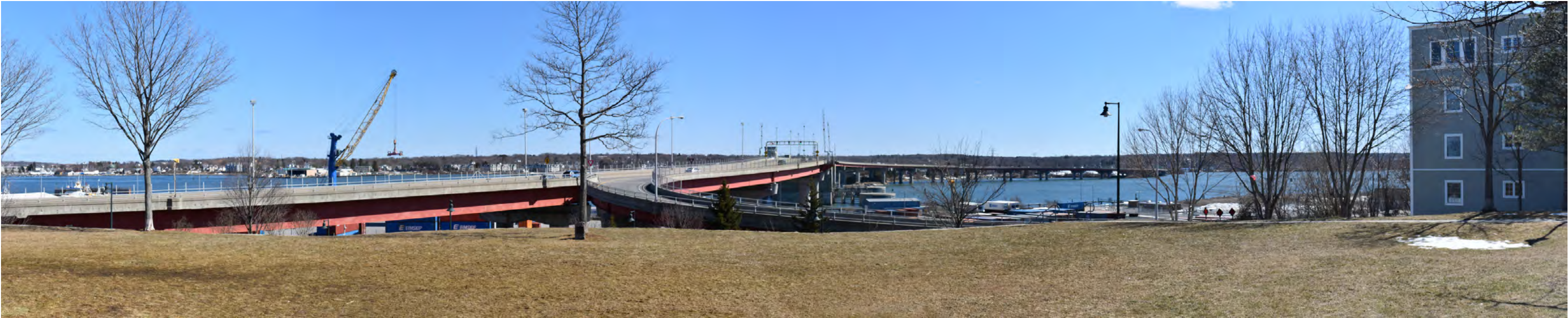
Existing Conditions panoramic view looking west to south from York Street north of Harbor View Memorial Park toward Casco Bay Bridge.
