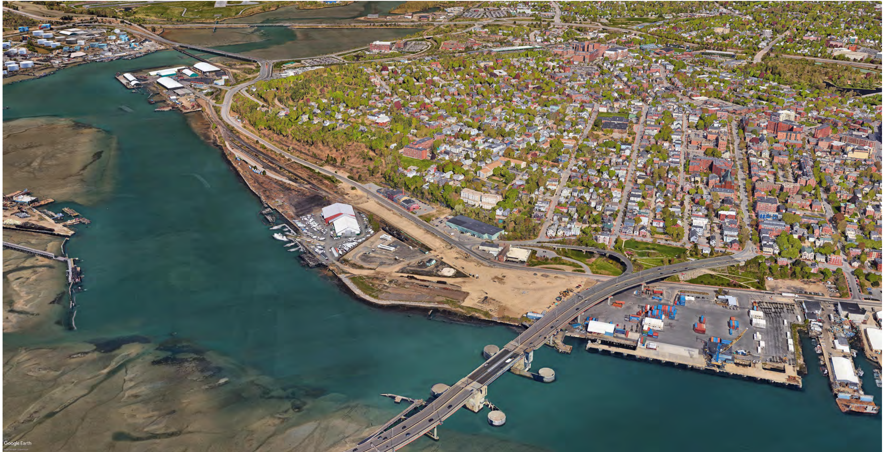
Existing Conditions bird's eye view looking west with Casco Bay Bridge in the foreground.
