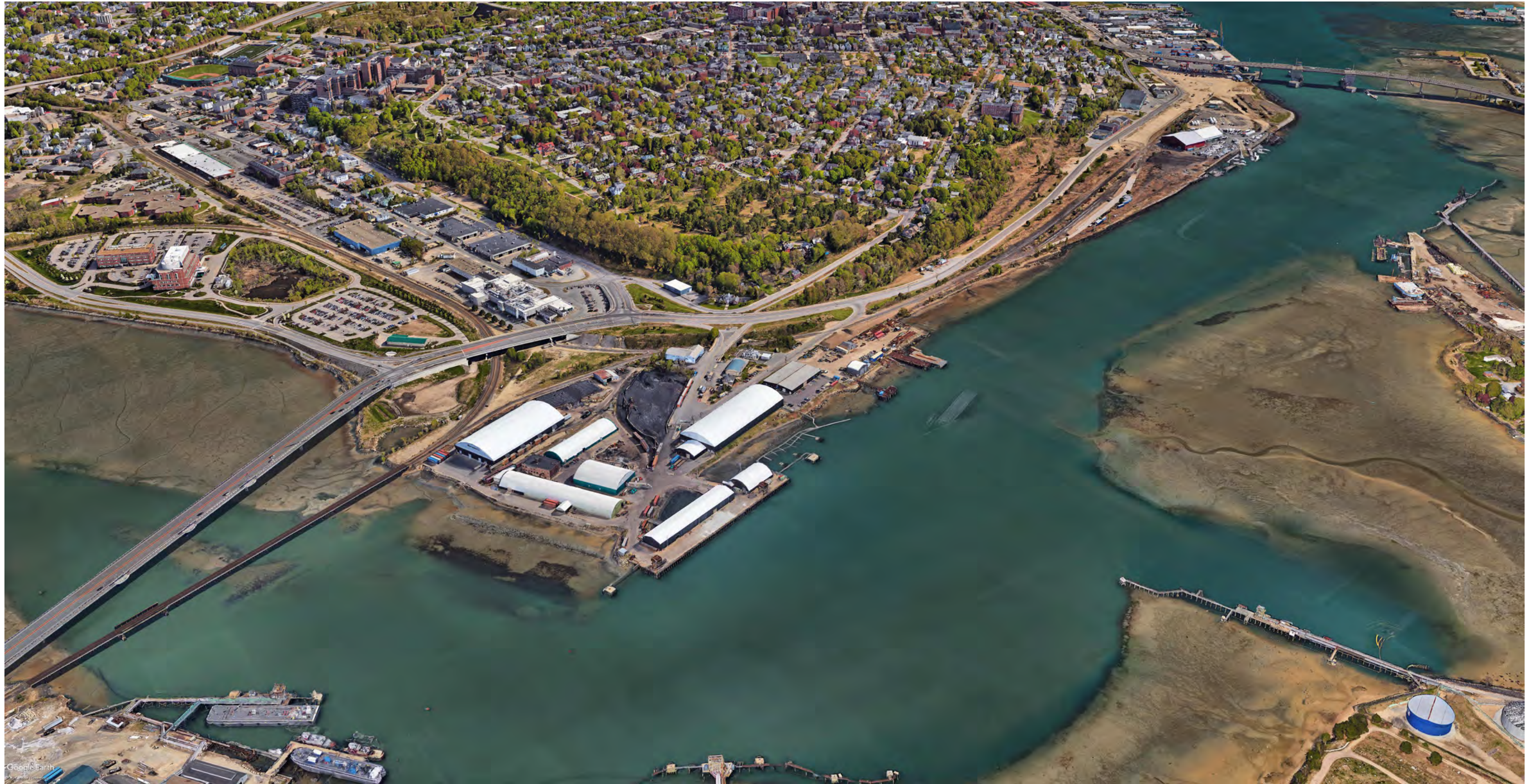
Existing Conditions bird's eye view looking east with Sprague Energy in the foreground.
