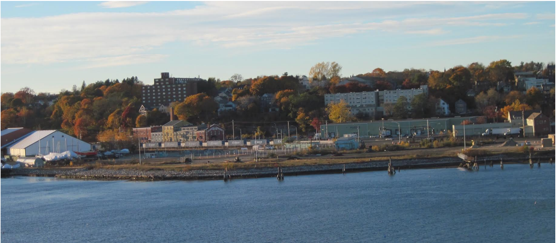
From Casco Bay Bridge
