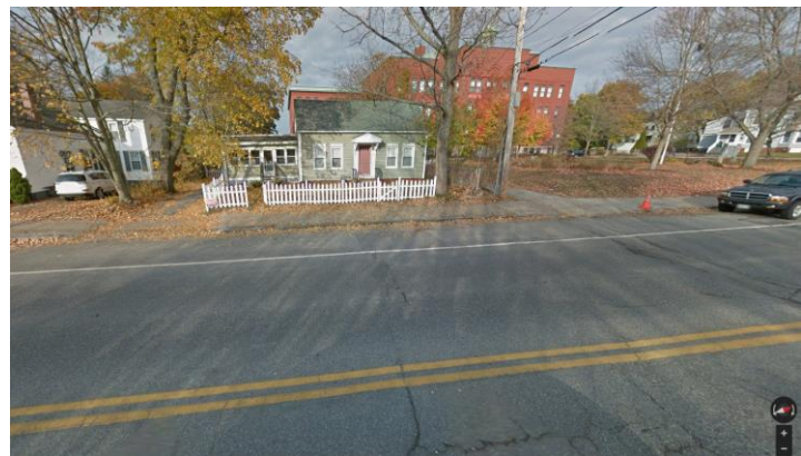
Figure 1: Existing Single-Family Structure
