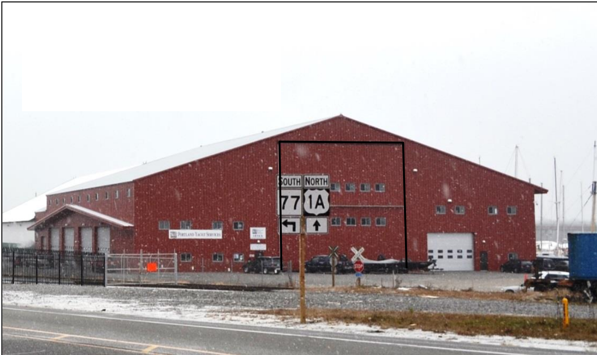
Figure 3: Boat Repair Shops Require Additional Height to Accommodate Larger Vessels
