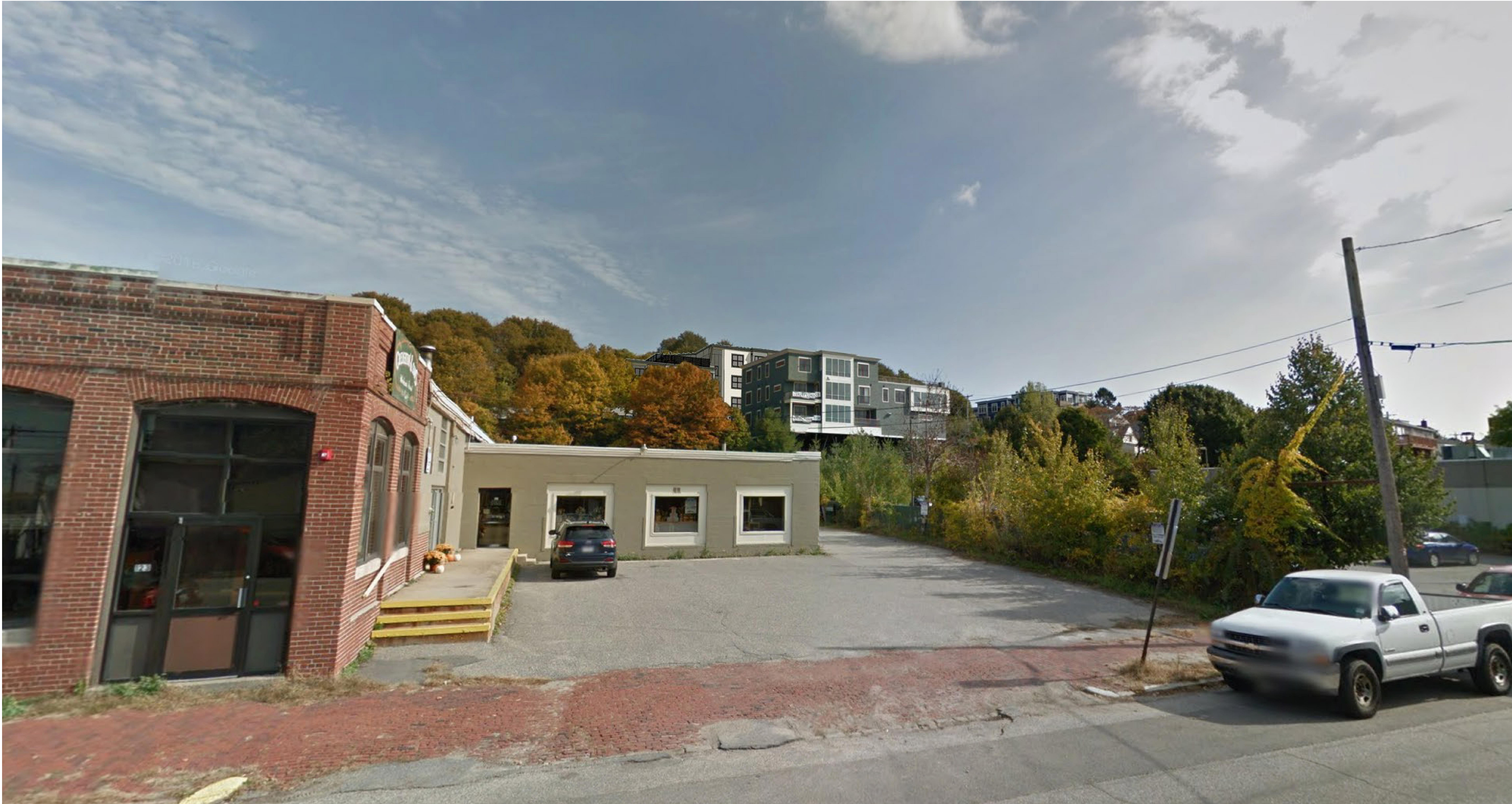
VIEW FROM WASHINGTON AVE.
