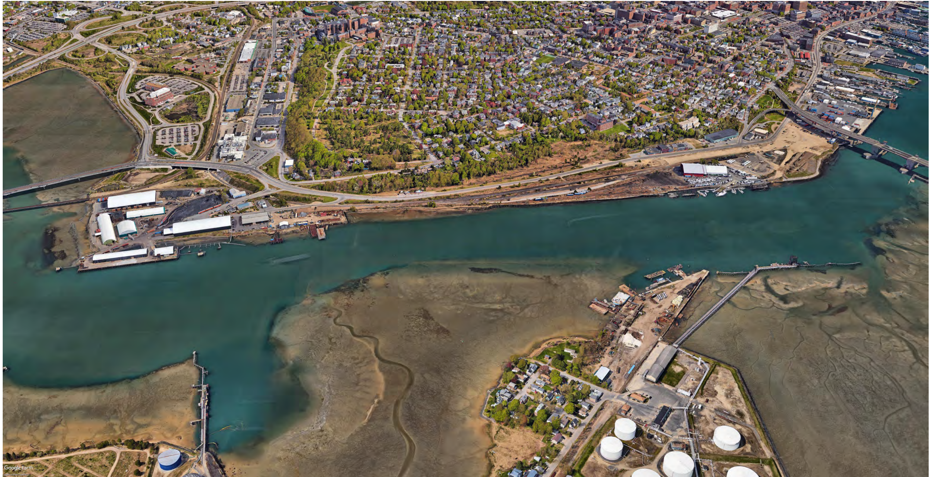
Existing Conditions bird's eye view looking north.
