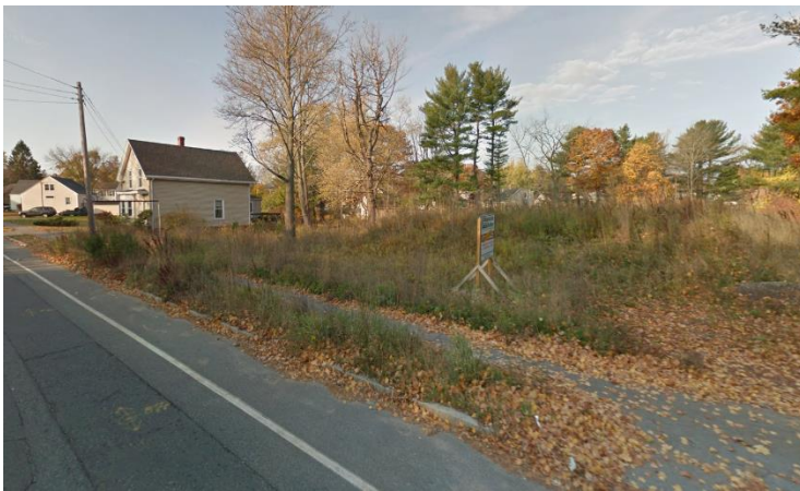
Figure 2: Existing conditions. Rise in elevation shows vegetated soil stockpile. Structure closest in view is to be demolished.
