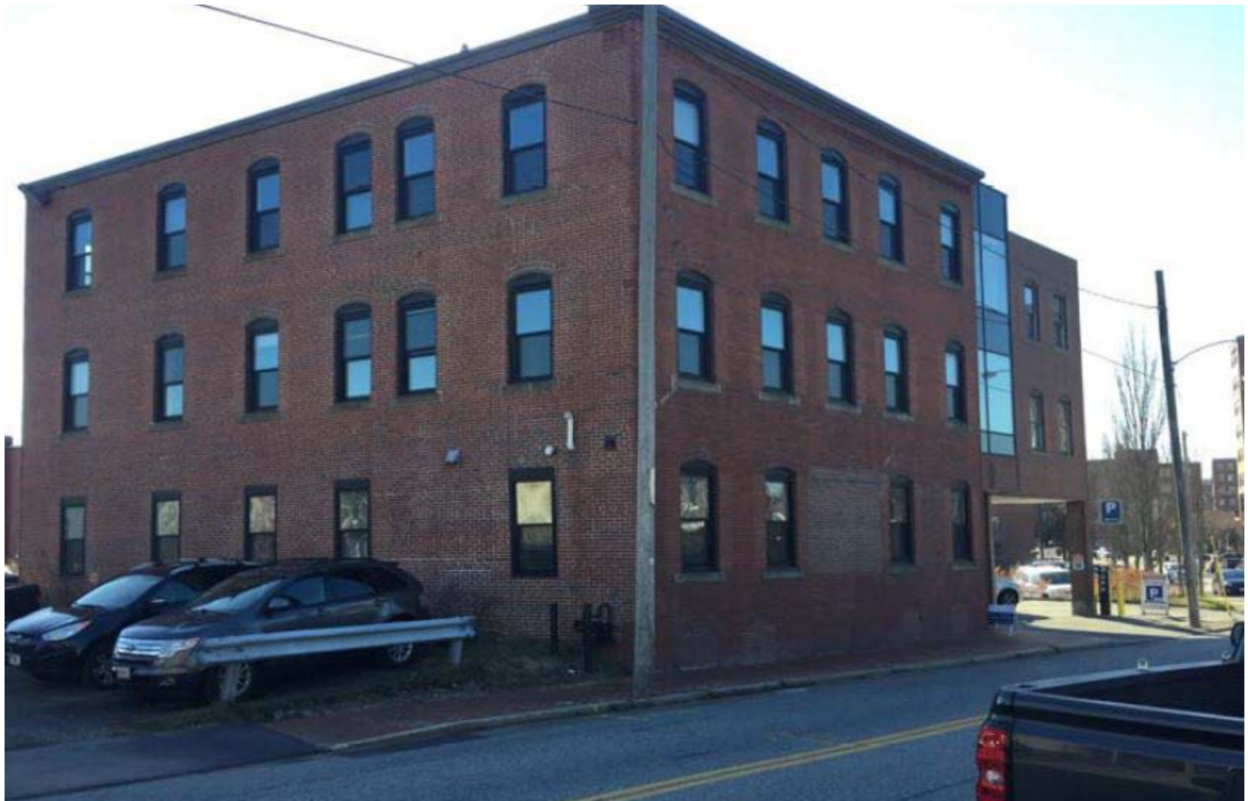
Existing condition of the site (image provided by applicant team)
