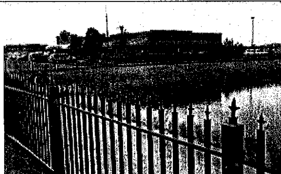
Photo 8: Fences have pros and cons as a safety measure; in general, do not rely exclusively on fencing for safety.
