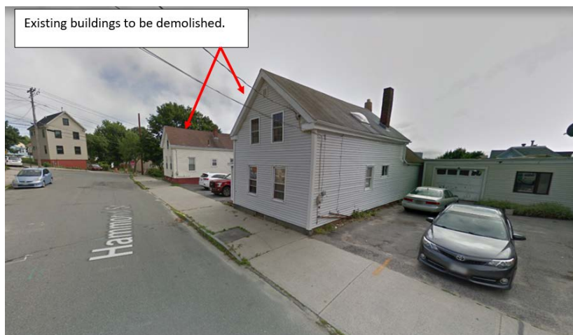
Figure 2: Existing conditions of site at Hammond Street frontage.
