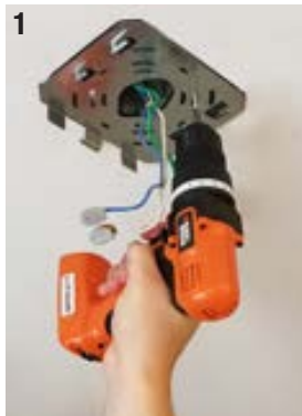
1 Mount plate to junction box.
