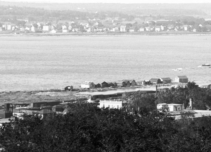
Back Cove before construction of Marginal Way – Looking northwest from Congress Street
