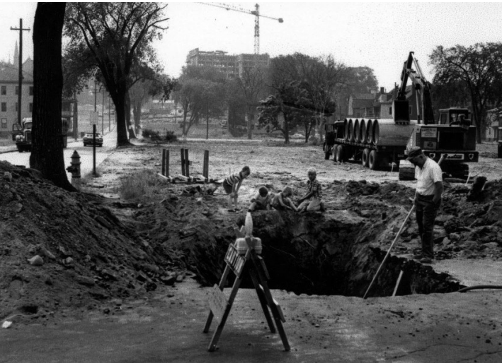
Construction of Franklin Arterial c. 1968 – Looking east from Marginal Way
