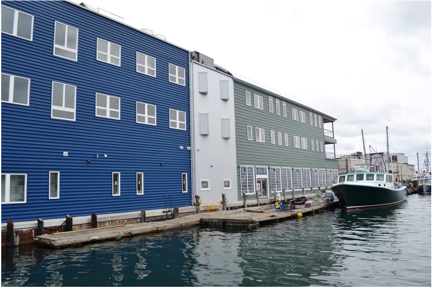
New Development at Maine Wharf, King Tide 2015
