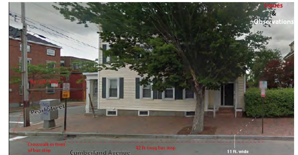
Figure 2-23: Existing conditions at a near-side stop, located at 255 Cumberland Avenue
