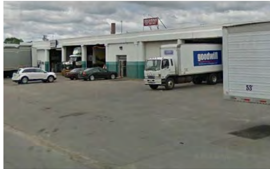
Figure 5-38: Fox Street before driveway improvements
