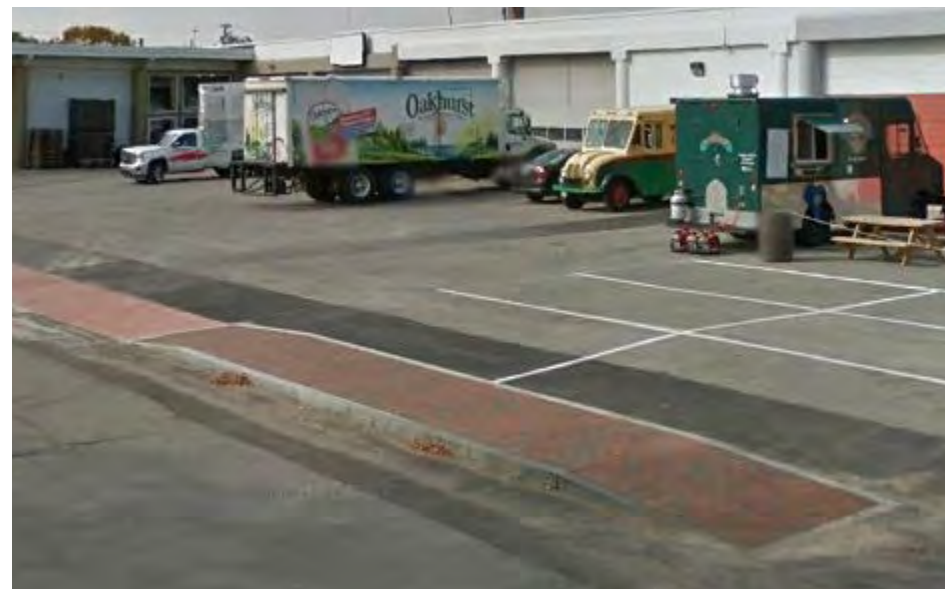
Figure 5-39: Fox Street after driveway improvements
