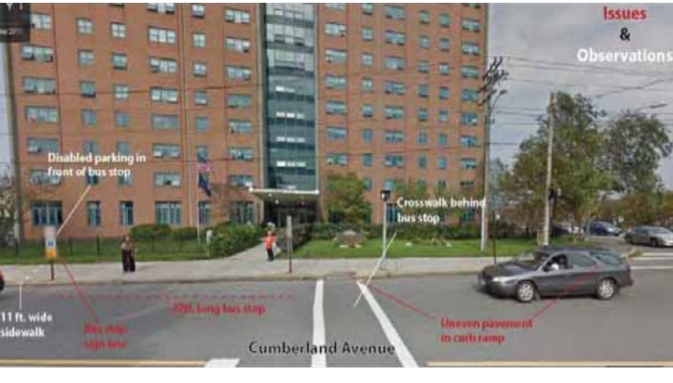
Figure 2-22: Existing conditions at a far-side stop, located at Franklin Towers on Cumberland Ave
