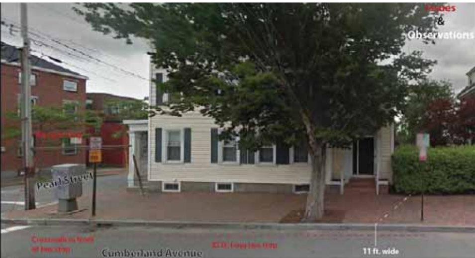
Figure 2-23: Existing conditions at a near-side stop, located at 255 Cumberland Avenue
