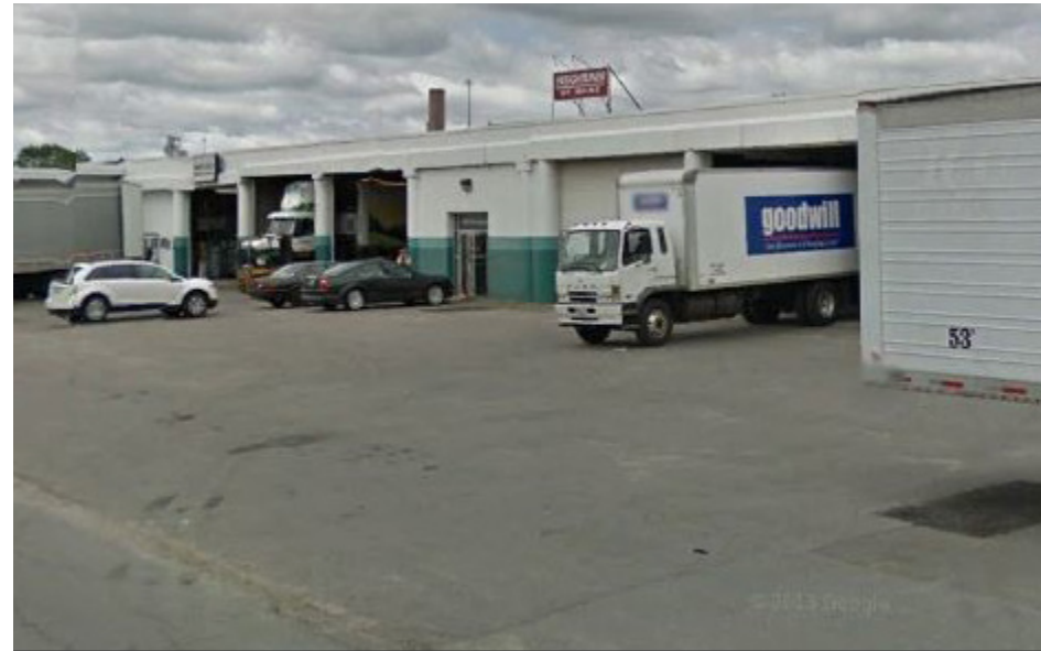
Figure 5-38: Fox Street before driveway improvements
