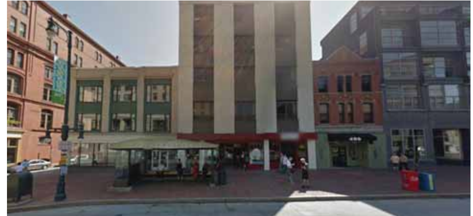
Figure 2-29: An existing bus stop that serves as a good example for Bayside is the Monument Square stop on Congress Street. This bus stop, located within a bus pull out, or bus bay, has sufficient length for buses to pull out of the travel lane and to the curb. Rider amenities include a shelter, bench, and trash receptacle. The sidewalk adjacent to the stop is 25 feet wide and provides a level landing area (five feet wide by eight feet deep area at the front door zone). Crosswalks with curb ramps are provided in close proximity to the stop.
