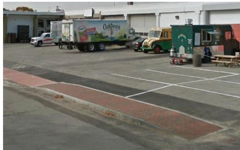
Figure 5-39: Fox Street after driveway improvements
