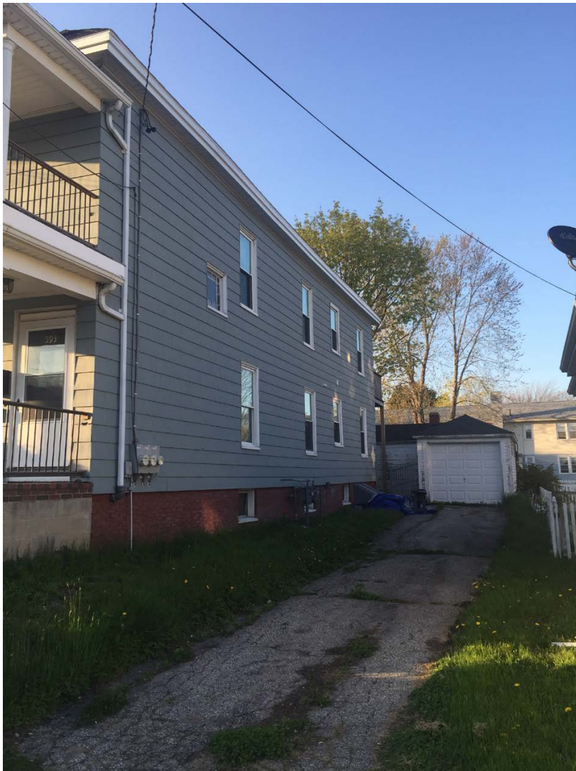
View from across washington Ave showing rear side of the house.
