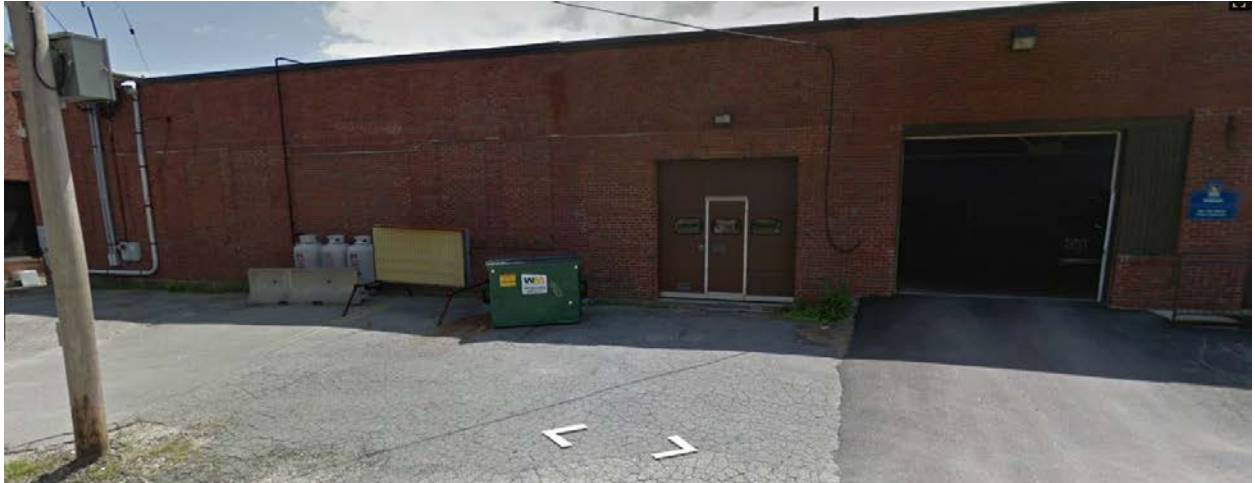
Rear of Property (Small overhead door)
