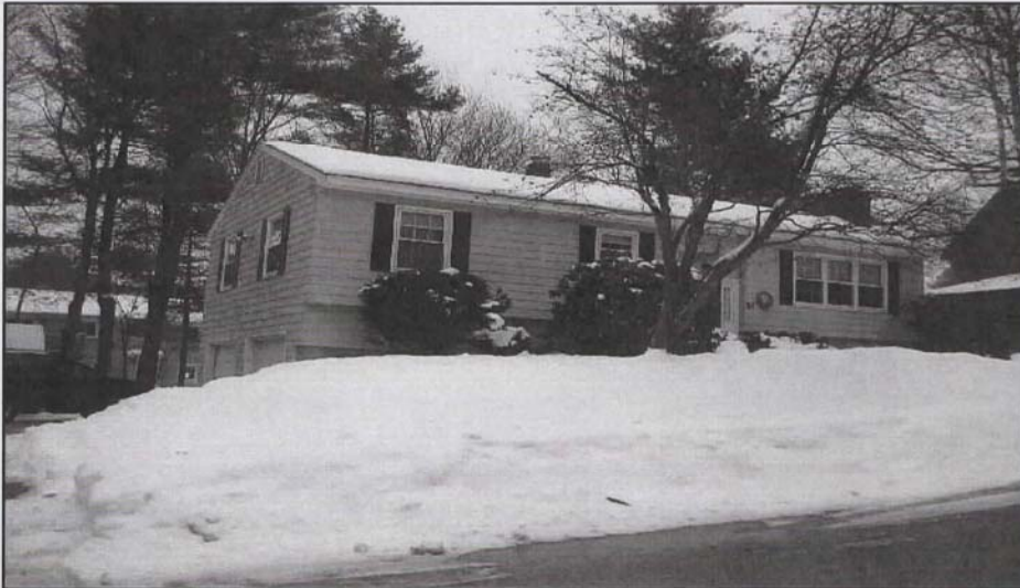
FRONT VIEW OF SUBJECT PROPERTY
