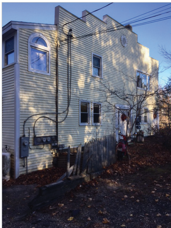
Front (street side)
