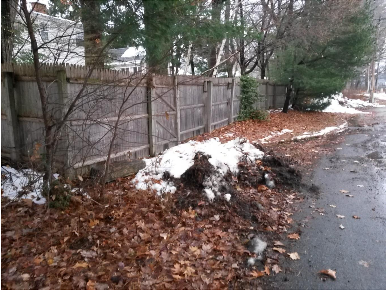
Lyseth Elementary School north property line opposite new gym addition – existing conditions Nov.2018
