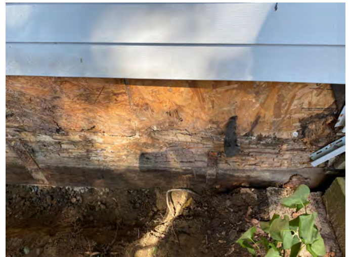
ADDITION EAST SIDE ROT
