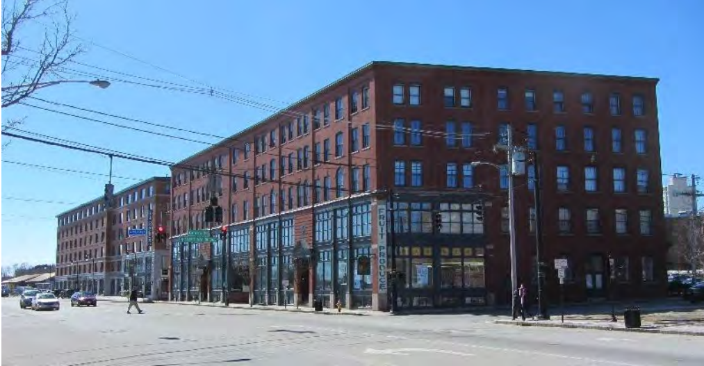
Figure 4: 1902 Porteous warehouse in foreground and new construction beyond.
