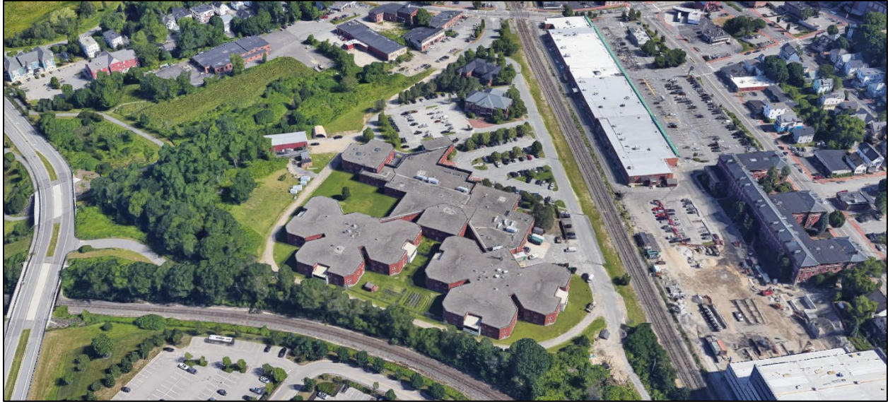
Figure 2: Aerial View of Site (facing north)
