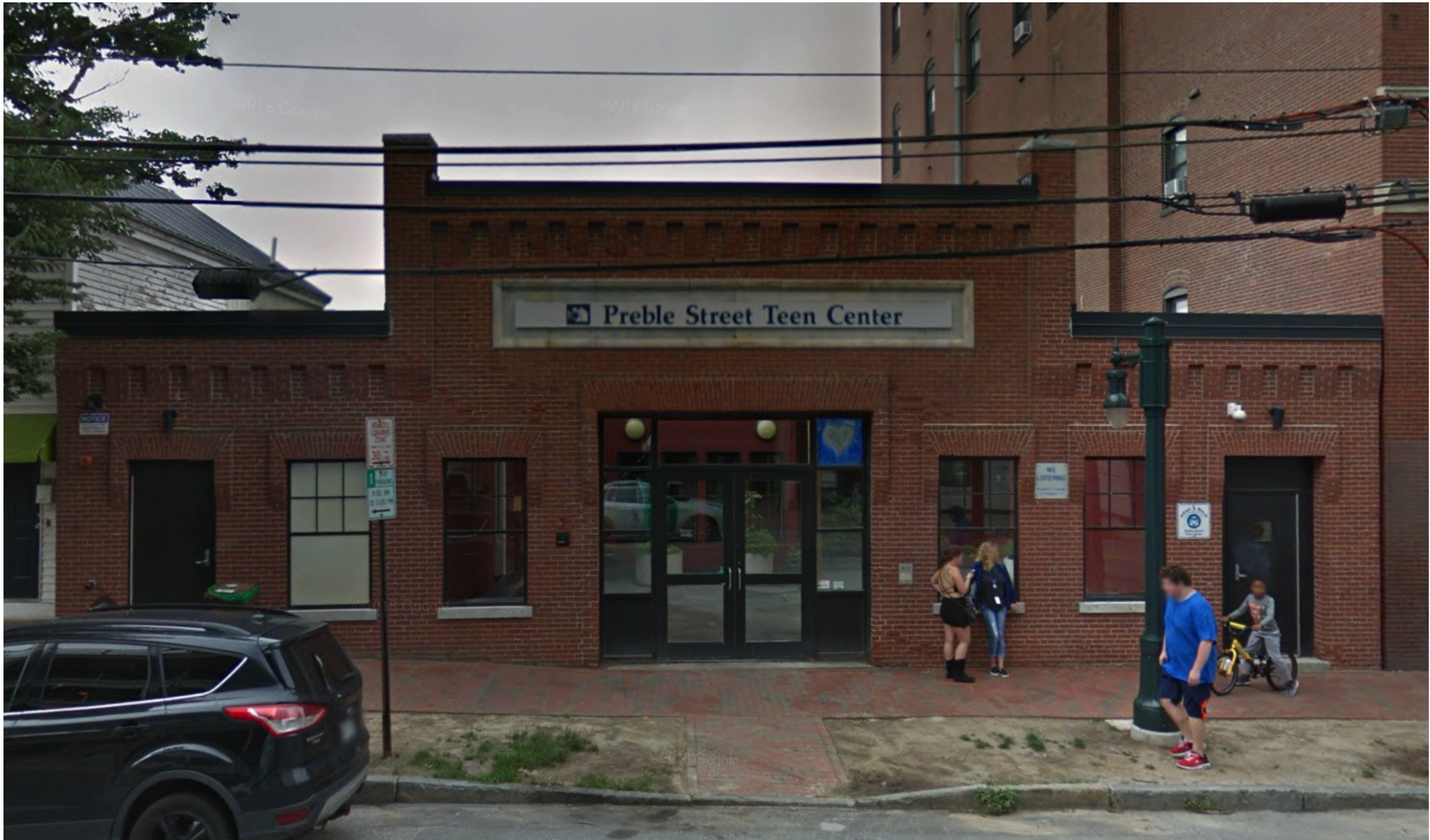
EXISTING CONDITIONS PHOTO
