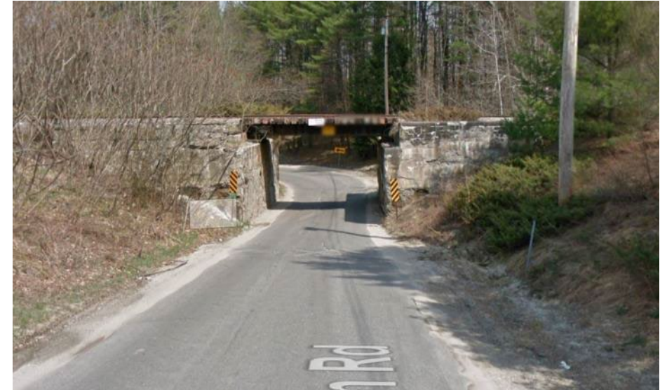
Berlin Subdivision bridge over Allen Road in Pownal
