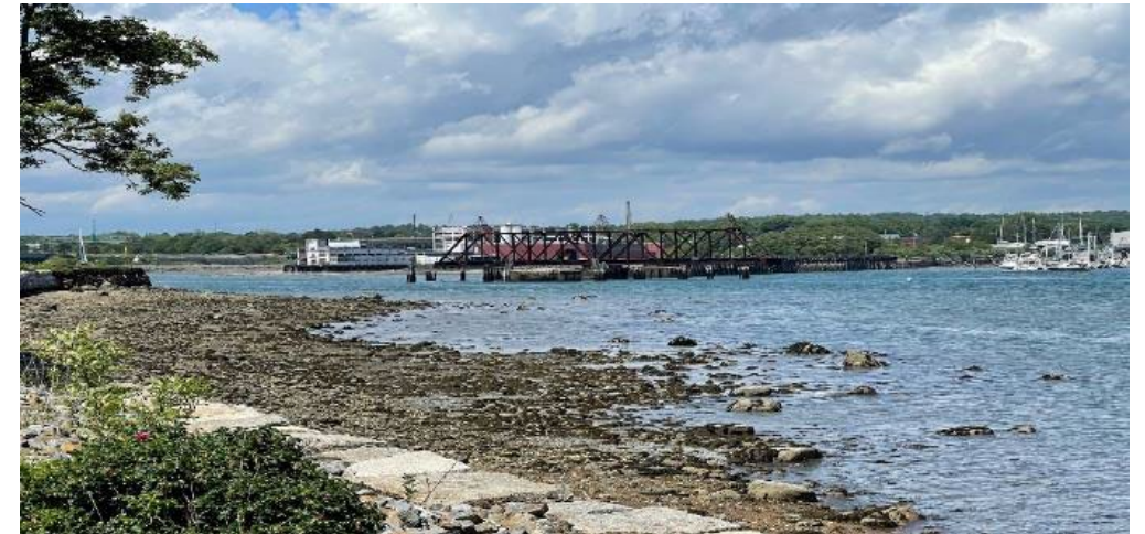
Back Cove Bridge in Portland
