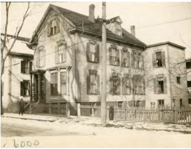
87 MUNJOY - 1924 TAX PHOTO 2 OVER 2 AT ALL WINDOWS
