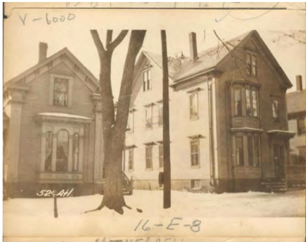
52 ATLANTIC - 1924 TAX PHOTO 2 OVER 2 AT ALL LARGE WINDOWS
