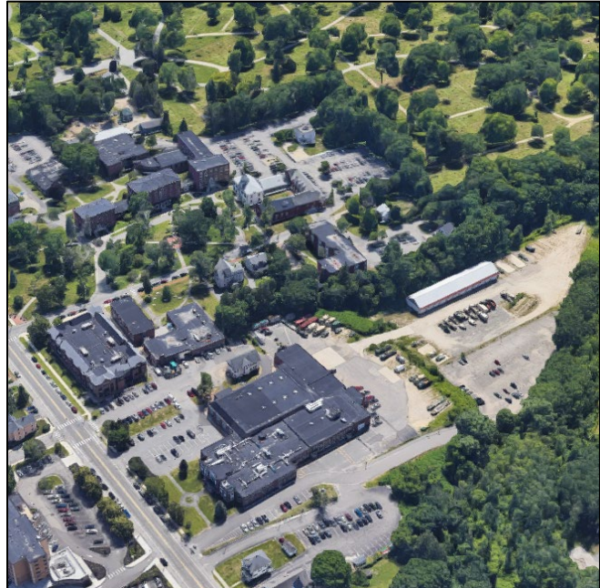
Figure 1. 780 Stevens Avenue in Campus Context
