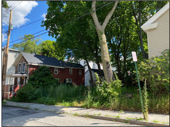
Figure 2. 31 Forest Street, Existing Conditions
