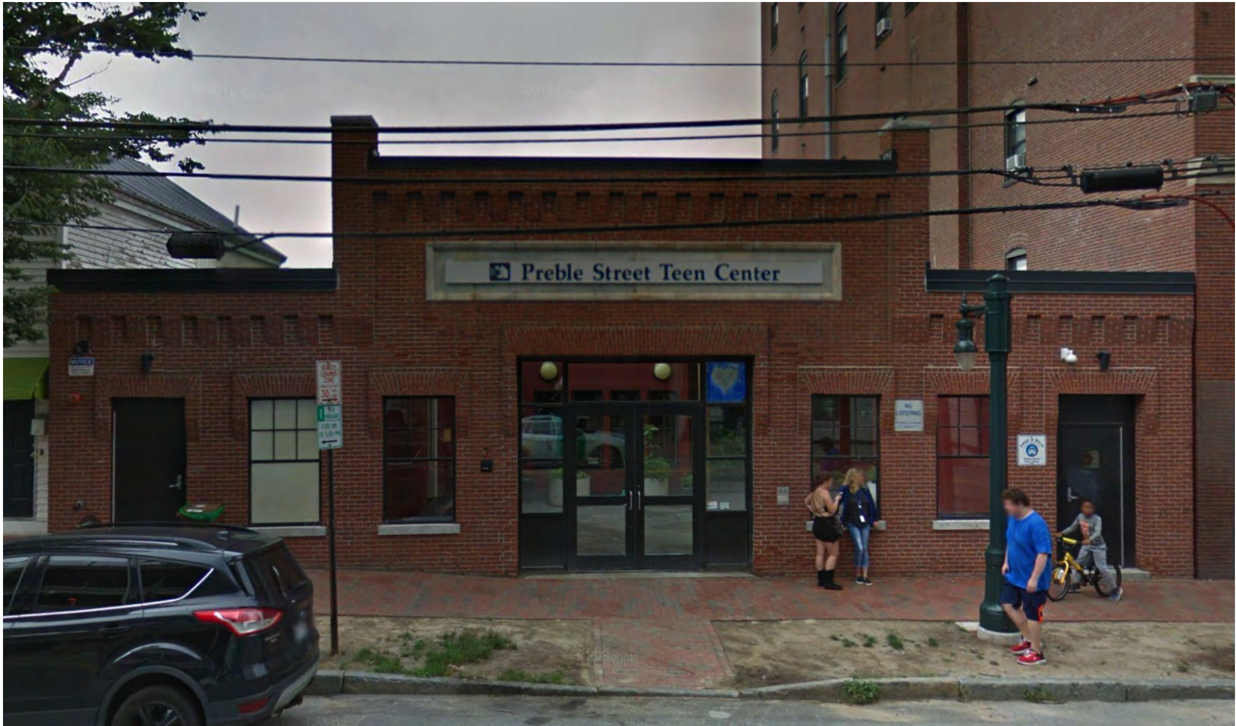
EXISTING CONDITIONS PHOTO
