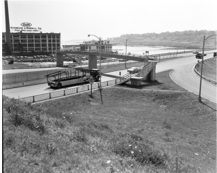
Figure 17: Image of former pedestrian bridge spanning over I-295 from the B&M Factory Site to the Southbound I-295 on-ramp at Washington Avenue. Source: MaineDOT
