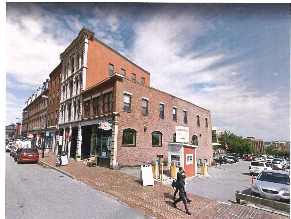
1 VIEW LOOKING EAST ON FREE STREET
