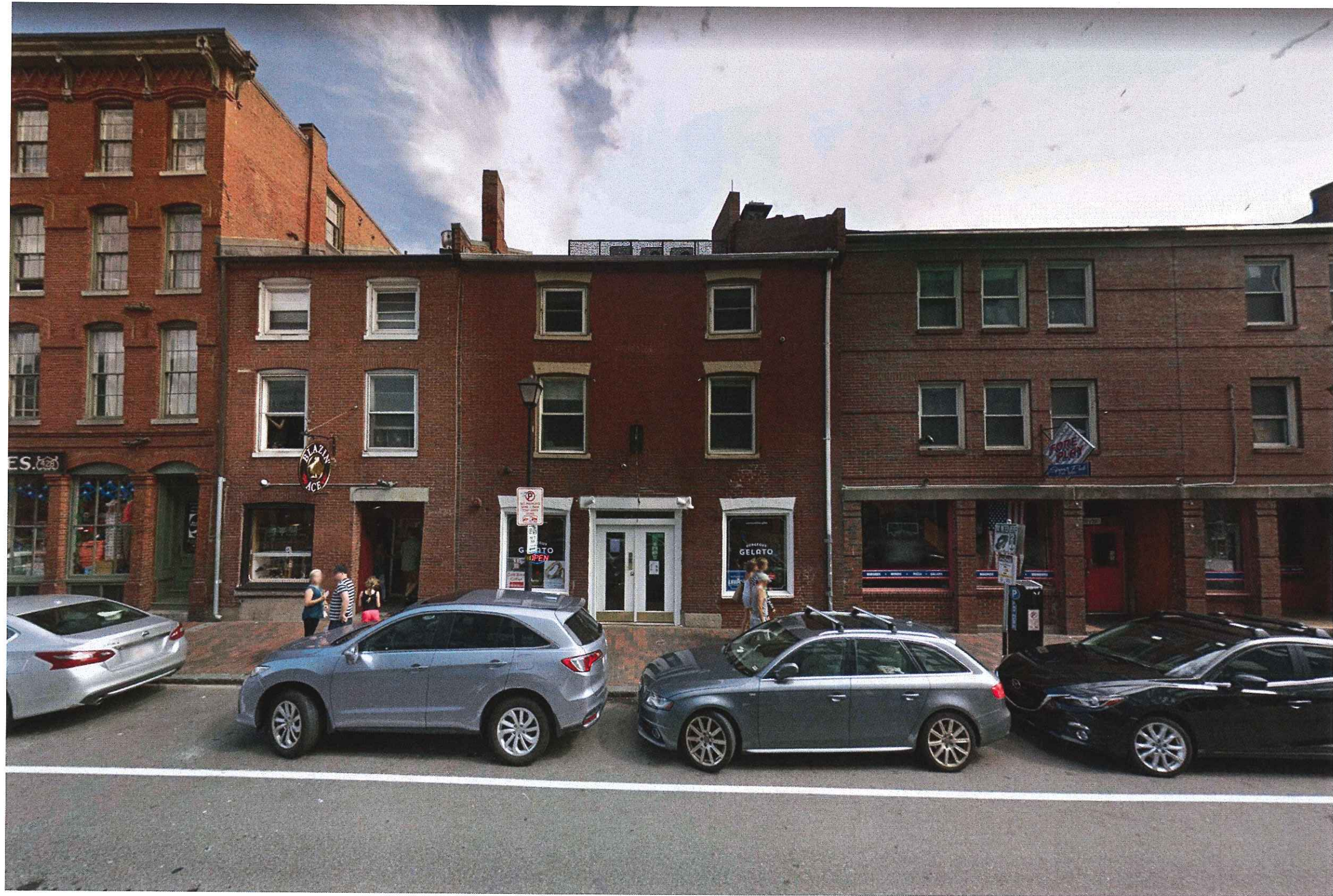
1 VIEW LOOKING SOUTH EAST ON FORE STREET N.T.S.
