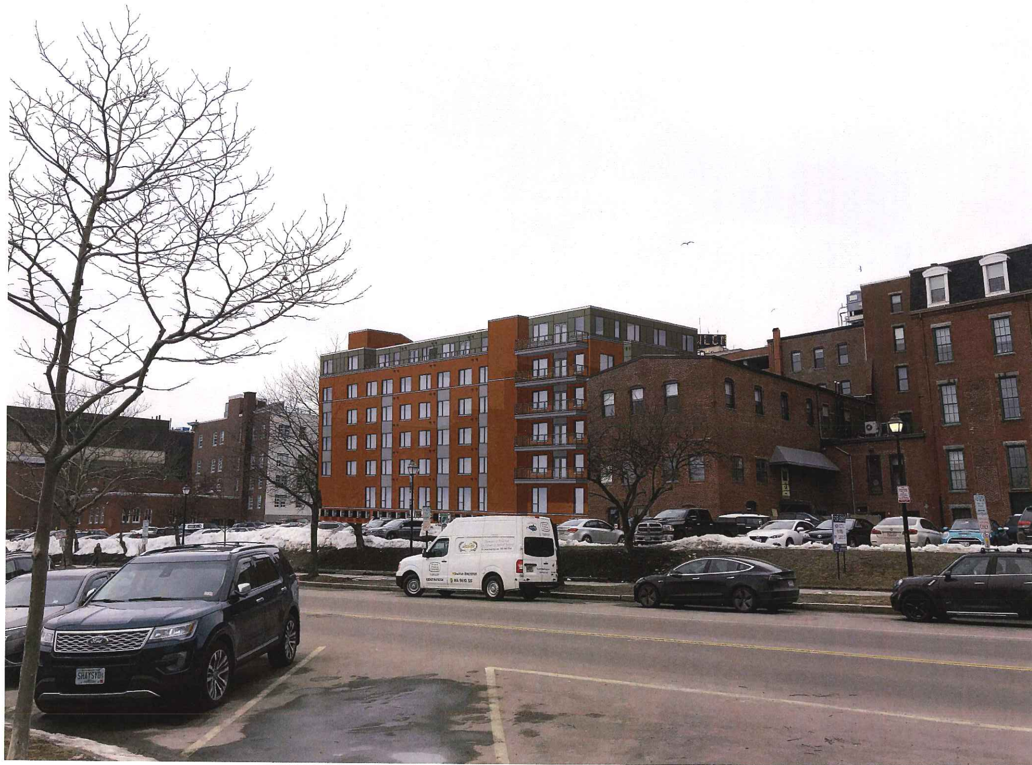
1 VIEW LOOKING WEST FROM SPRING STREET
