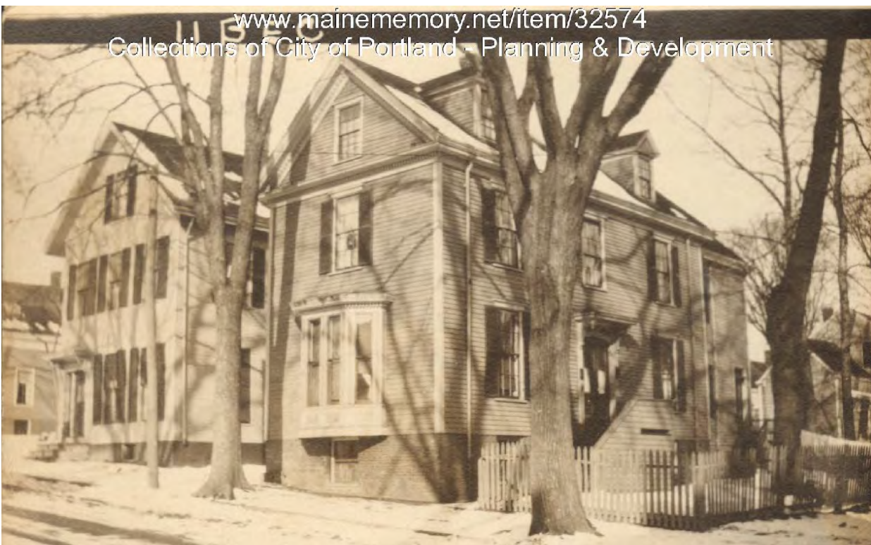
Figure 2: 1924 Tax Assessors photo of 11 O'Brien (then 9-11 Beckett Street).
