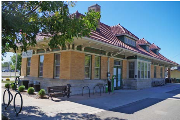
Figure 15: C&O Station in Muncie, IN. The Station is bounded by an active freight line and the Cardinal Greenway and currently serves as offices for the Cardinal Greenway. A similarly scaled building could provide retail, restaurant, and/or commercial support for a multi-modal station at 43 Sherwood Street under a B-5 zoning designation, but not under the current R-3 zoning.
