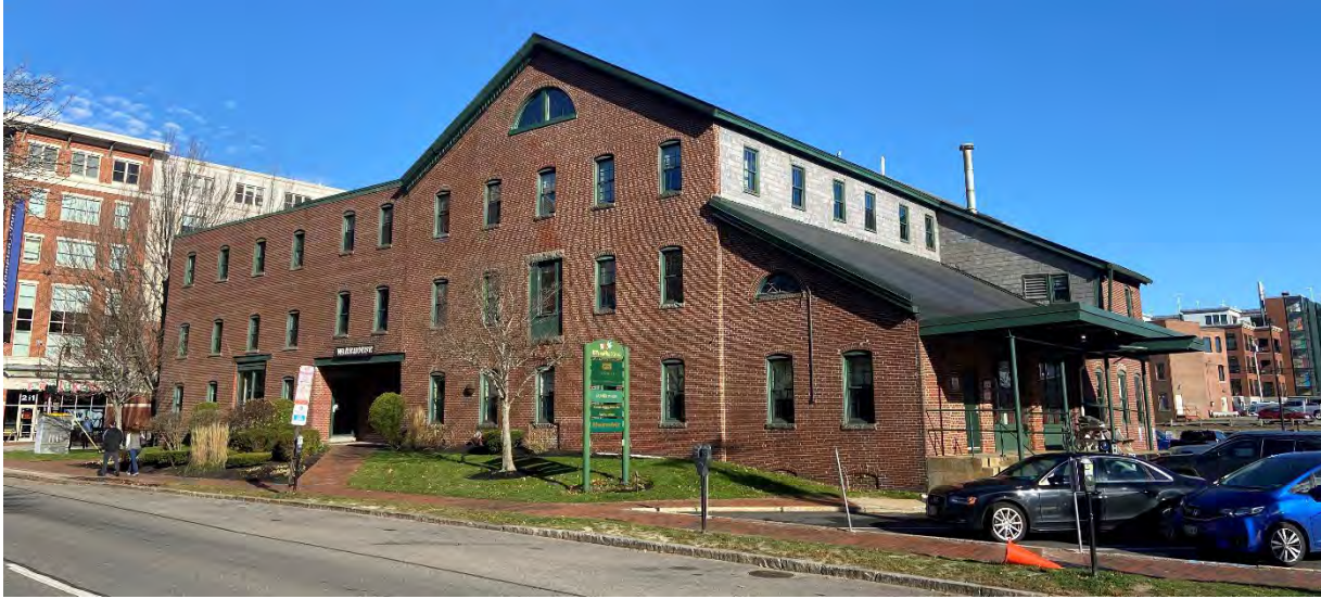
Figure 6: The Burnham & Rumery Cannery building located north of the Galt Block.
