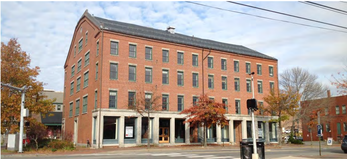
Figure 5: The Galt Block with the Burnham & Rumery Cannery beyond to the left, and the side of the Workingmen's Club to the right.
