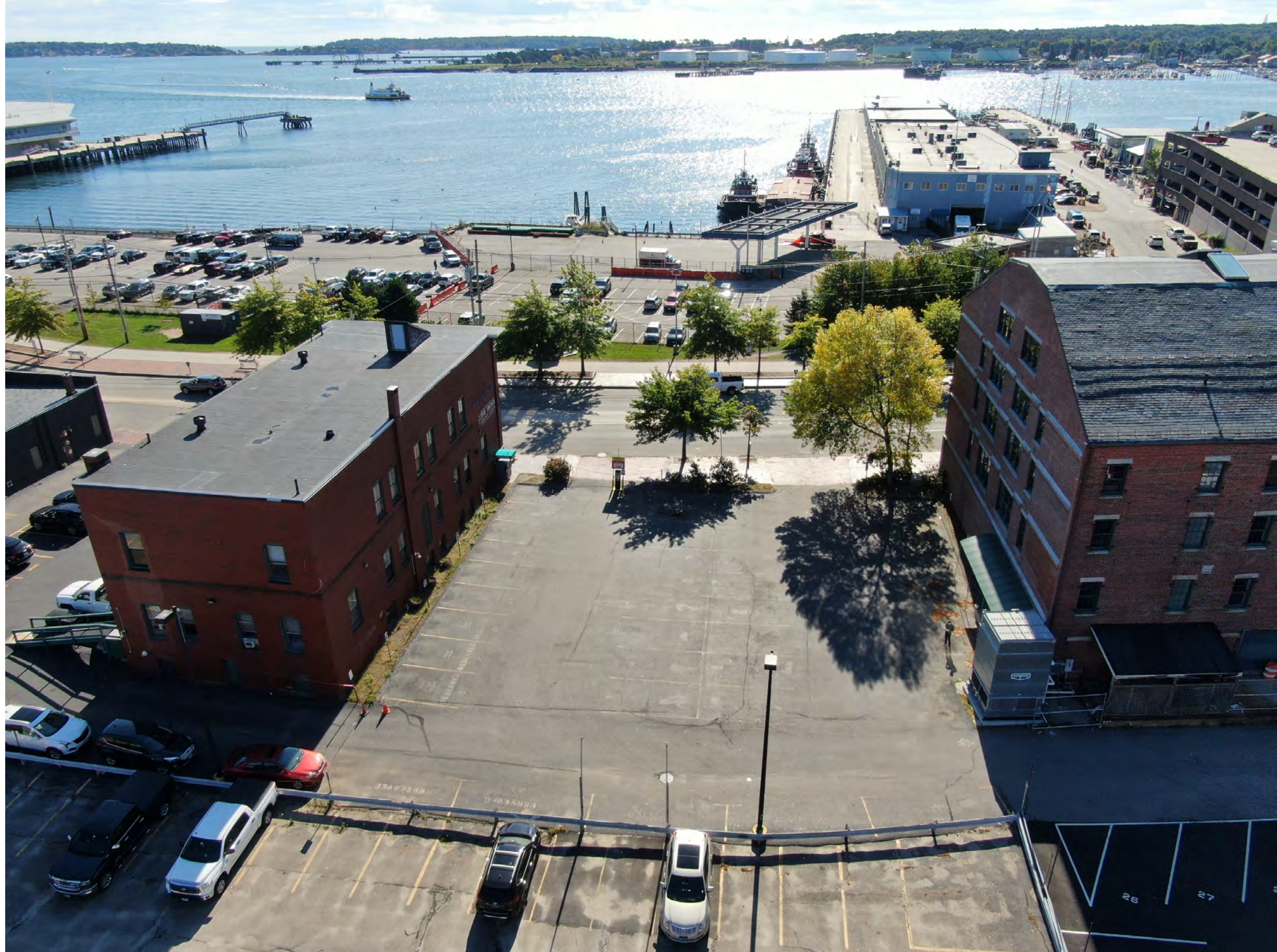
Current Site Conditions
